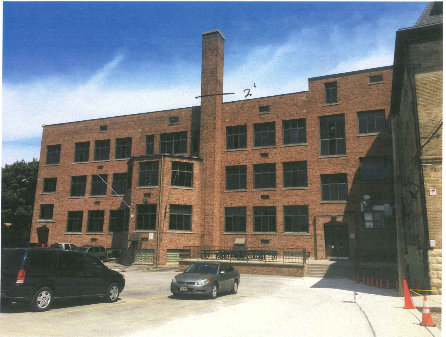
SCHOOL WEST ELEVATION OF CHIMNEY
