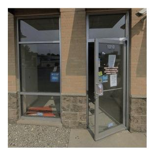
In addition to changing the existing door to a fixed panel, the proposal would include the application of an opaque film to the back of the storefront glazing, represented by squares on the elevation, to accommodate the program requirements of Exam Rooms 1, 2, and 3.
