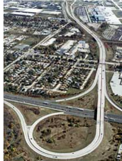
Aerial view of WIS 119 (Airport Spur) to General Mitchell International Airport in Milwaukee.
