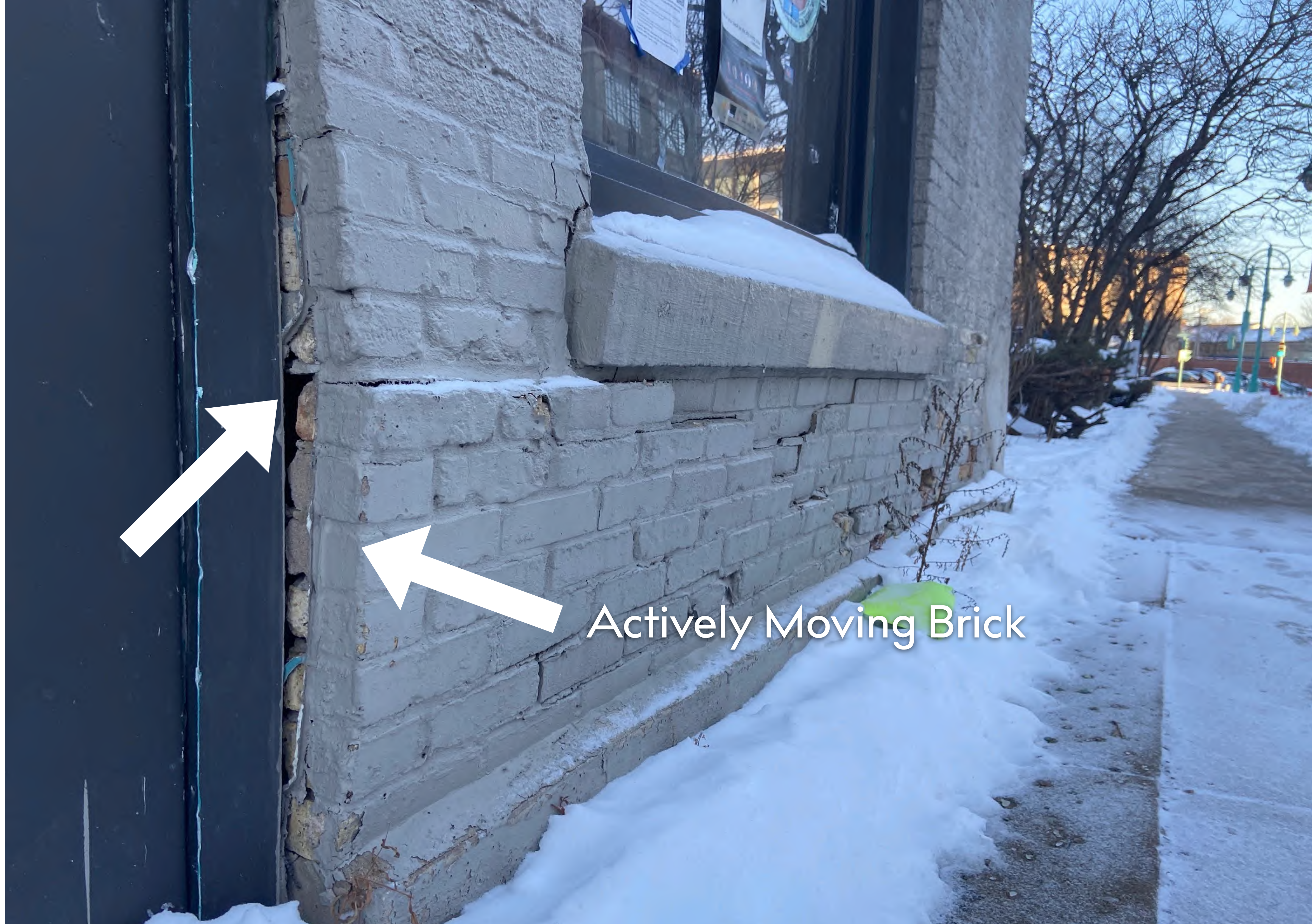
Structural Brick Deterioration
