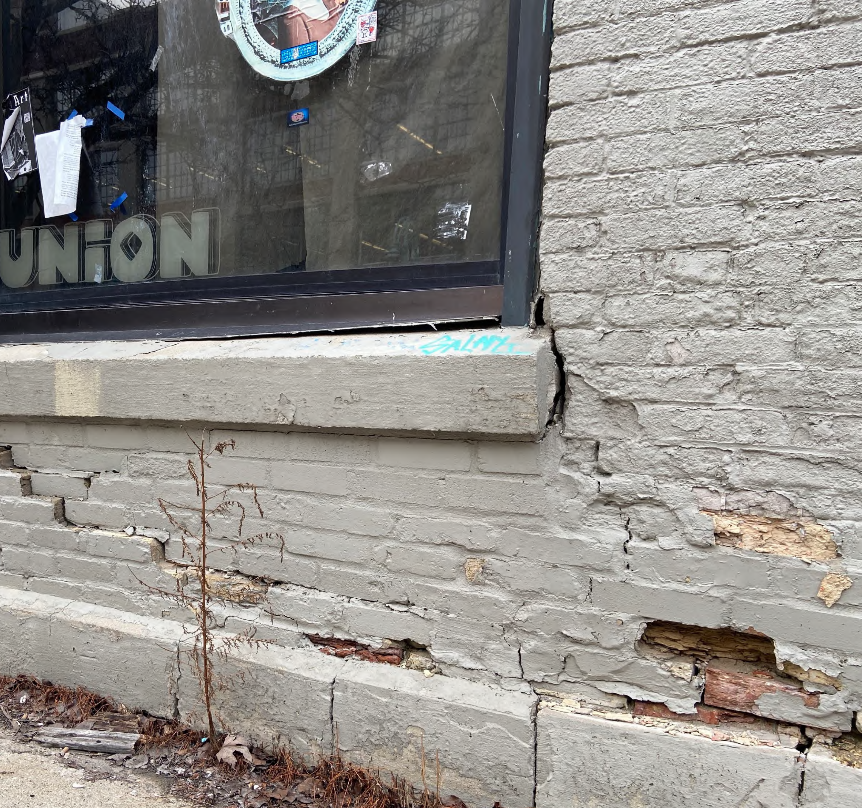
Structural Brick Deterioration
