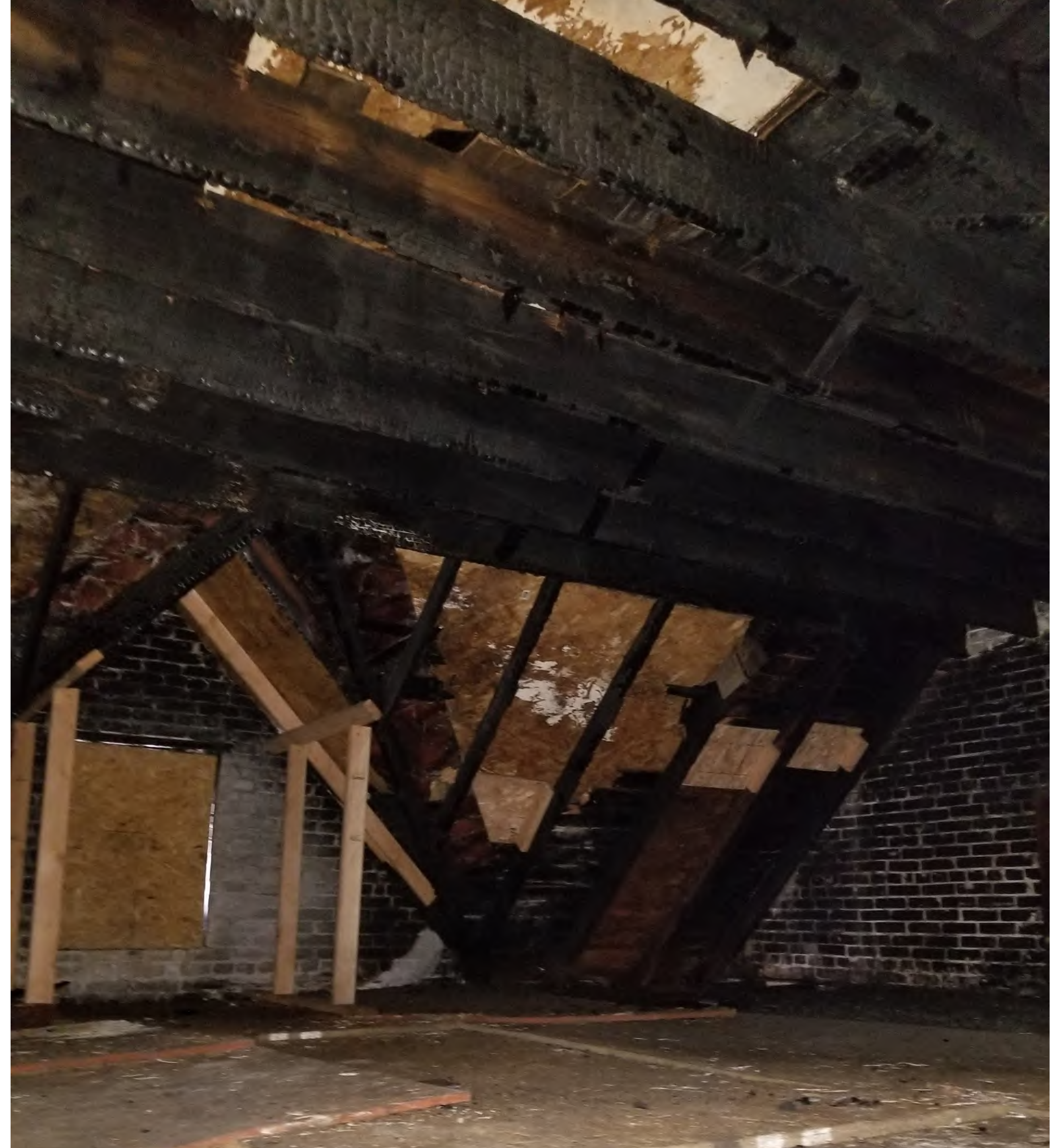
Roof - Structural Fire Damage
