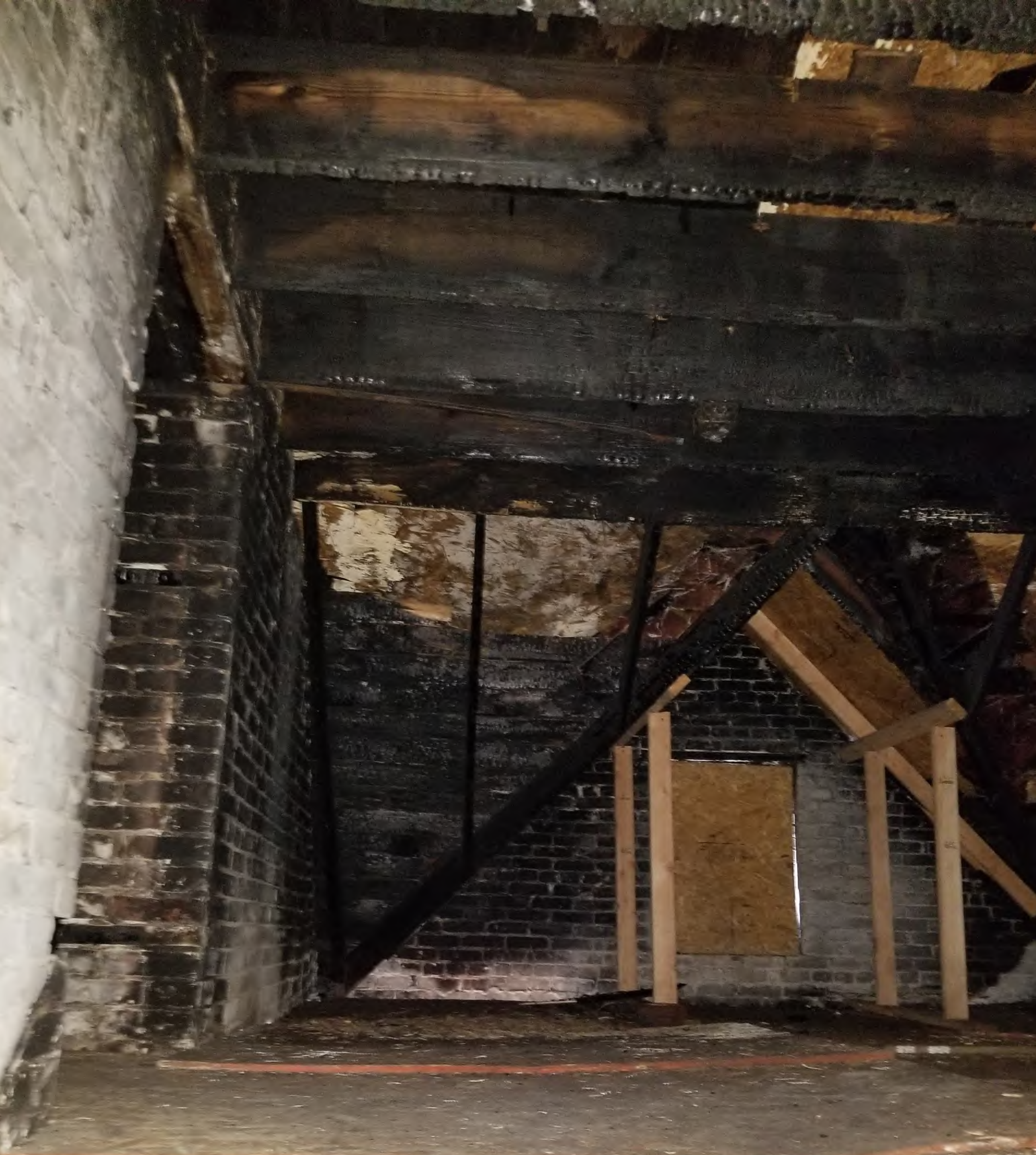
Roof - Structural Fire Damage
