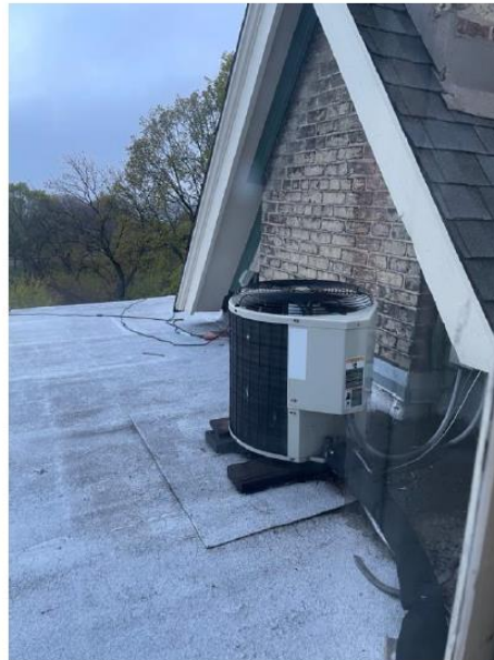
Rooftop with existing condenser:
