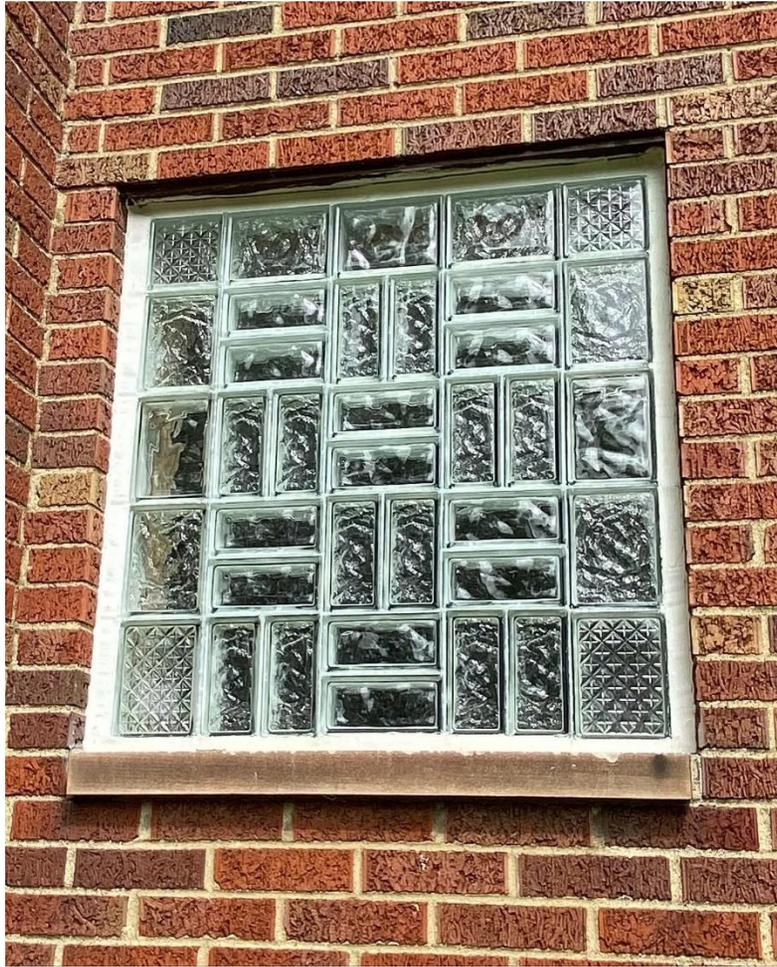
**Example of CORRECT glass block window installation. The blocks must be recessed from the surface of the exterior wall.**
