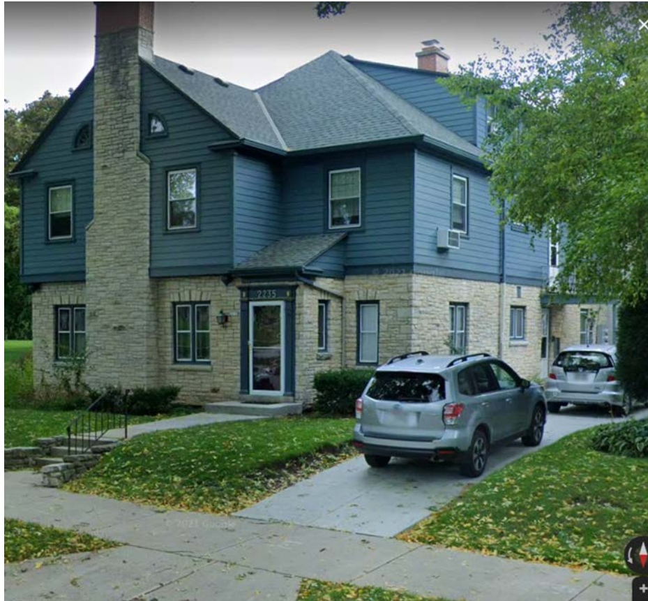
Existing porch visible
