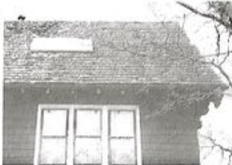
Current condition of roof. No rafter tails will be removed. Skylight can be removed on this elevation if desired.
