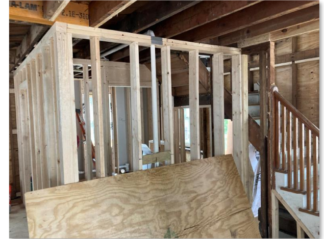
4423 N 25 th Street – Interior Framing
