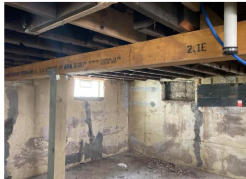
4423 N 25 th Street - Basement
