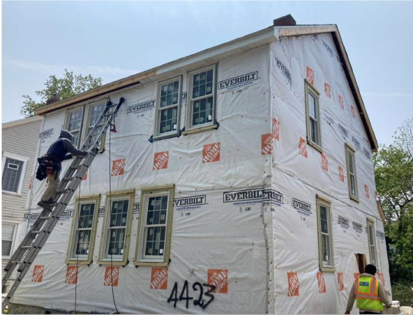
4423 N 25 th Street – Back Elevation
