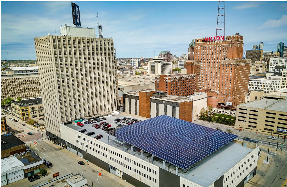
Clark Building Solar Canopy
