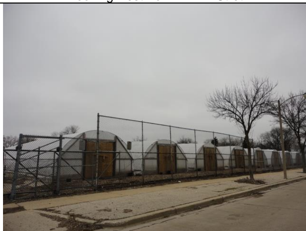
Looking westerly from N. 41 st Street
