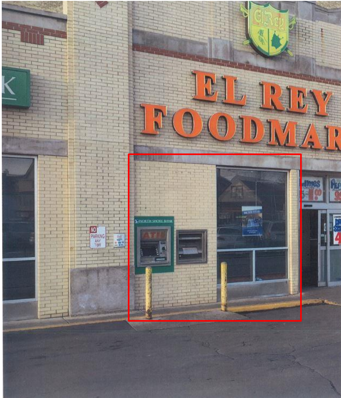
South Façade indicating area to be replaced with new brick
