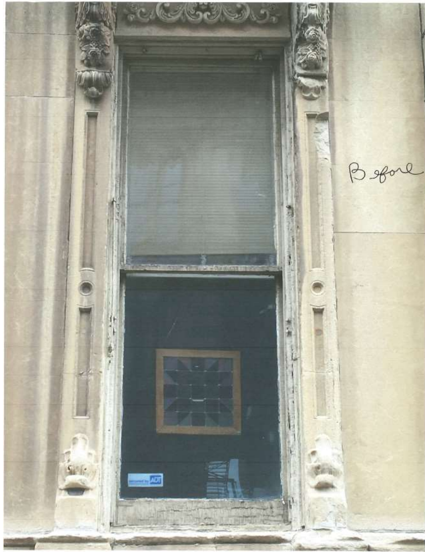
Typical "before" window
