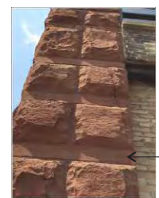
MOUNTING PLATES MUST ATTACH IN AREA BETWEEN BLOCKS
