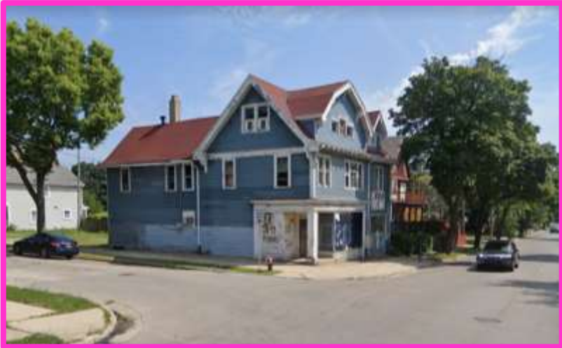
View from E Burleigh St looking northeast
