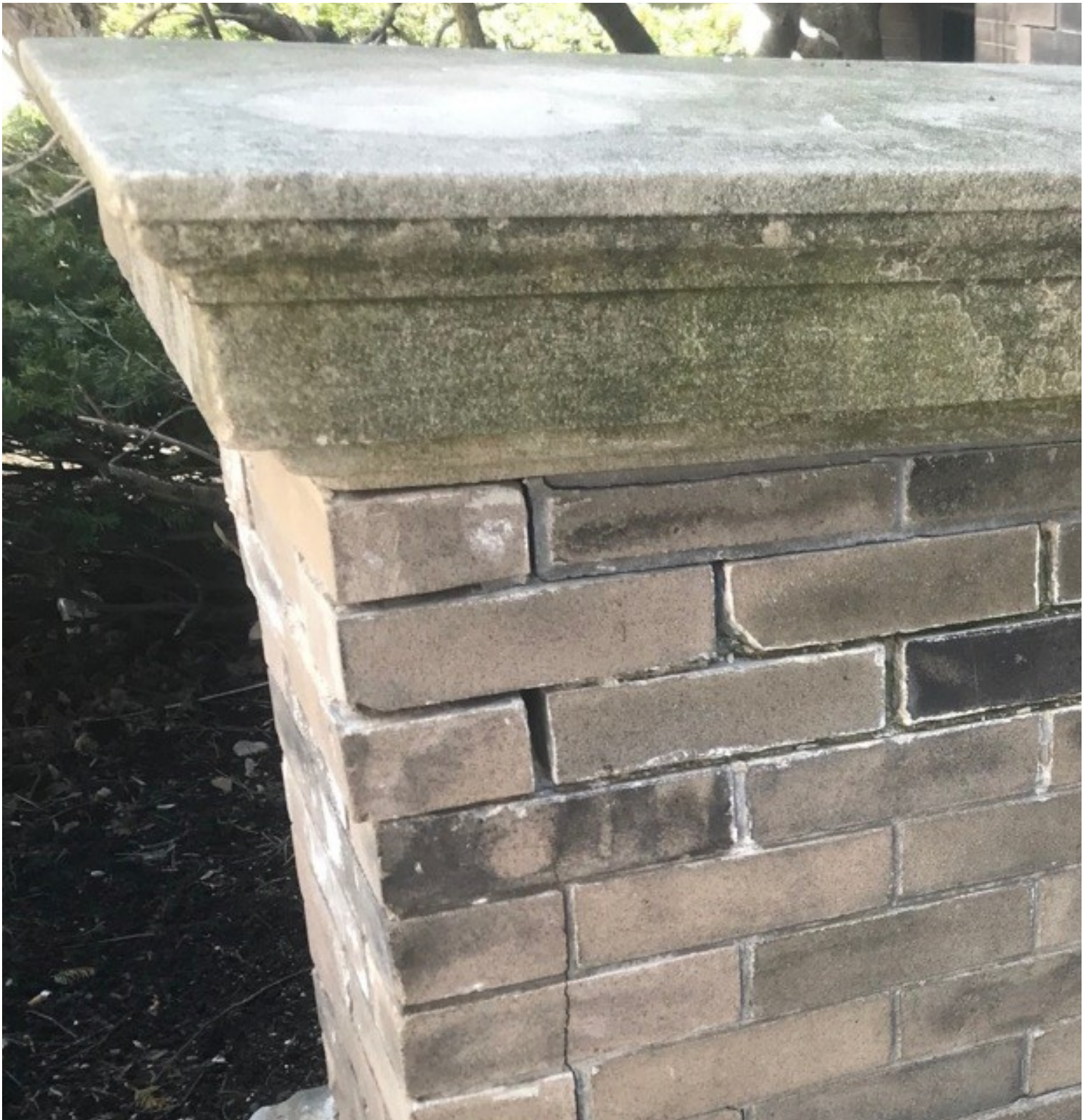
S front / interior face, again, I hand displaced those bricks, could pull them out entirely. Mortar gone.
