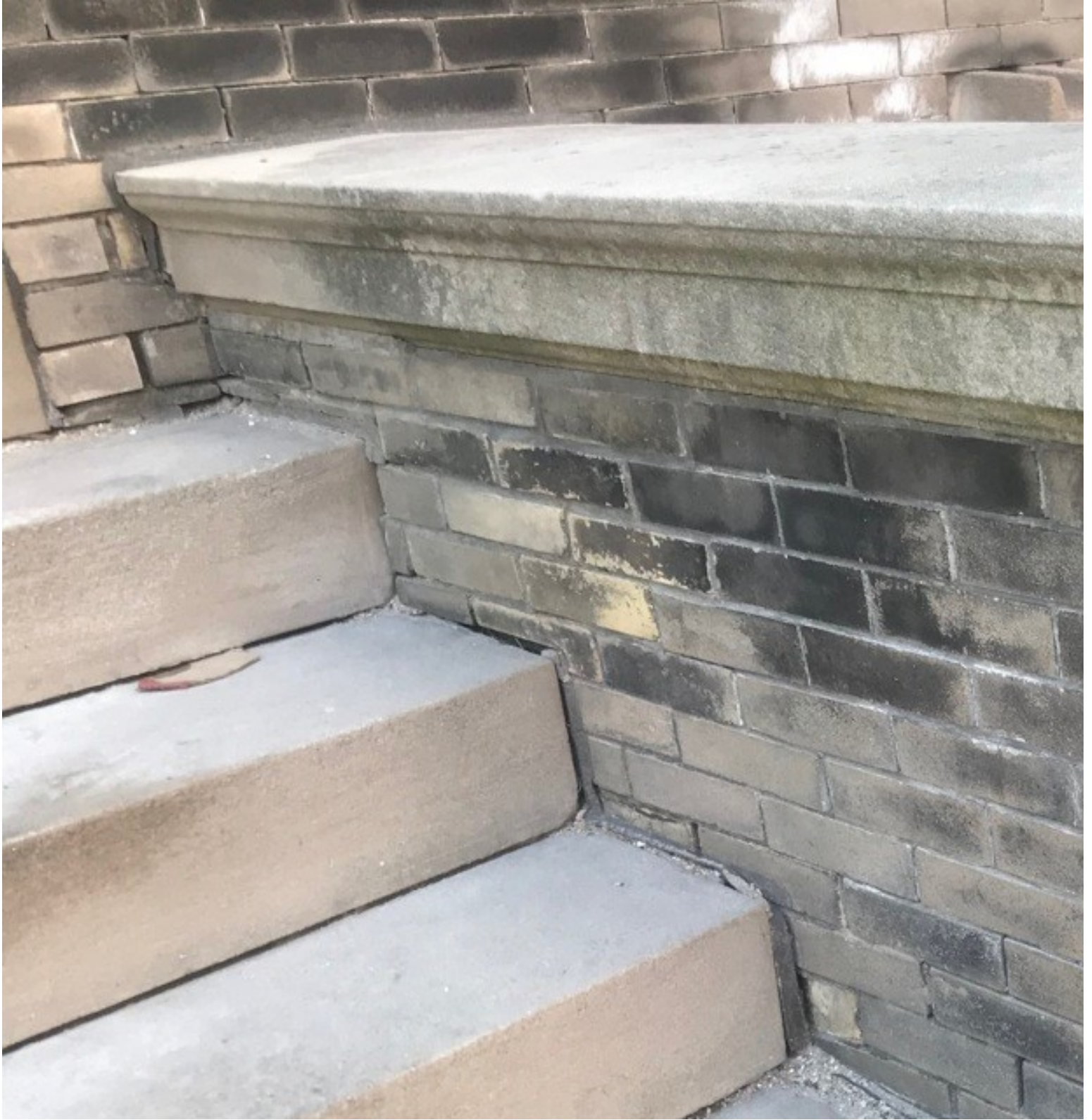
N interior face
