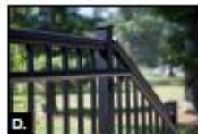
Handrail and Guardrail Material: Matte Black powder-coated aluminum railing system with ADA handrails at the new stair going up to the second level. This stair starts 11'-1" behind the front face of the existing building.
