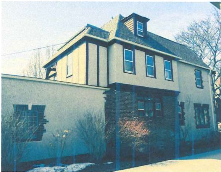
Side of house – looking south
