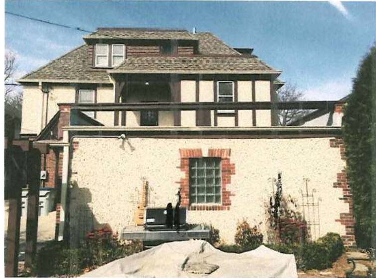
Back of house – looking west
