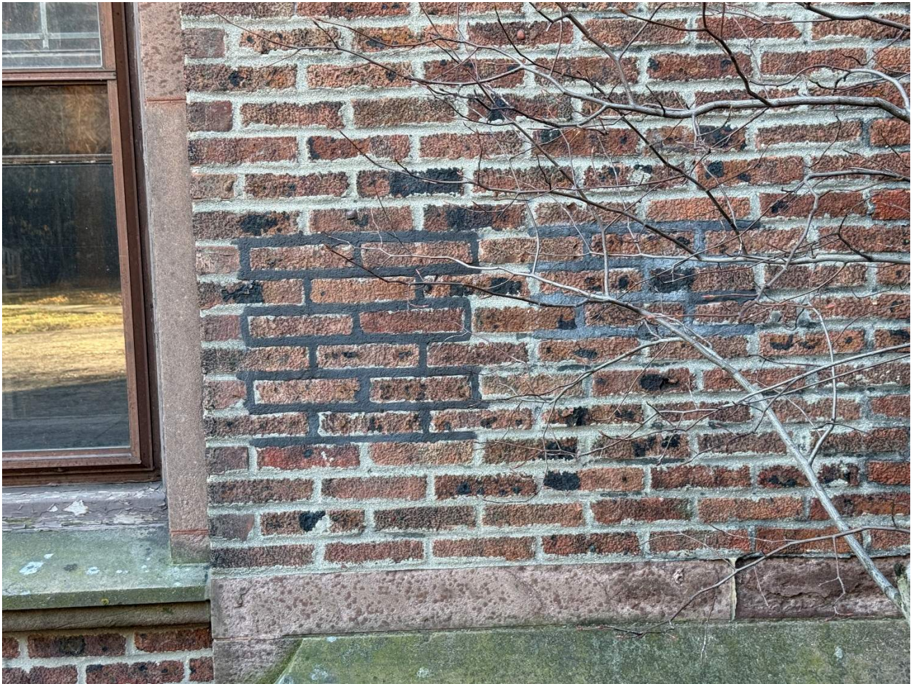
~2016 Mortar Mockup with original pigment (left):
