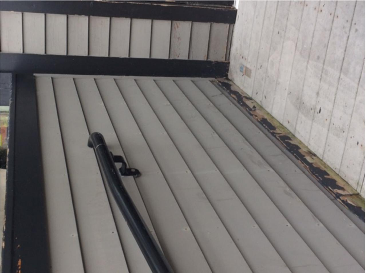
Existing landing area for ADA access to restaurant. Opening to be made to deck at landing, beyond existing hand rail. Deck to be level with landing.
