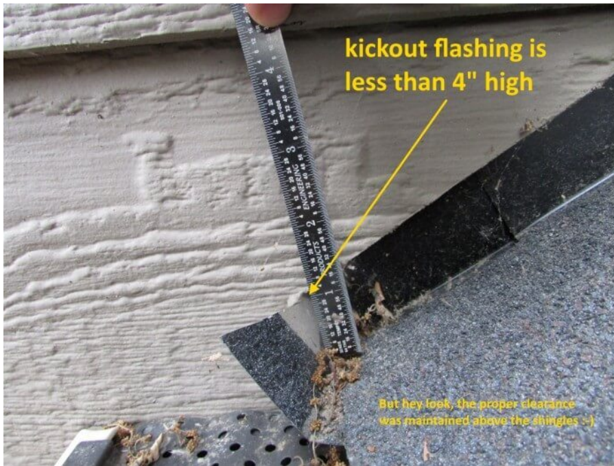
( http://www.structuretech1.com/wp-content/uploads/2015/09/Kickout-flashing-too-short.jpg )
