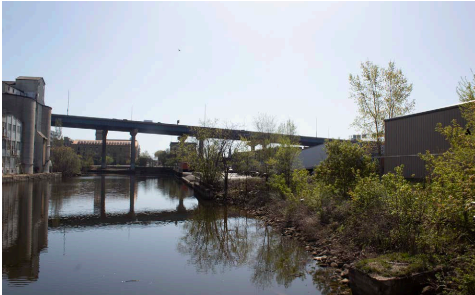
Image above shows the view from the 11th Street bridge over the Burnham Canal, looking east.
