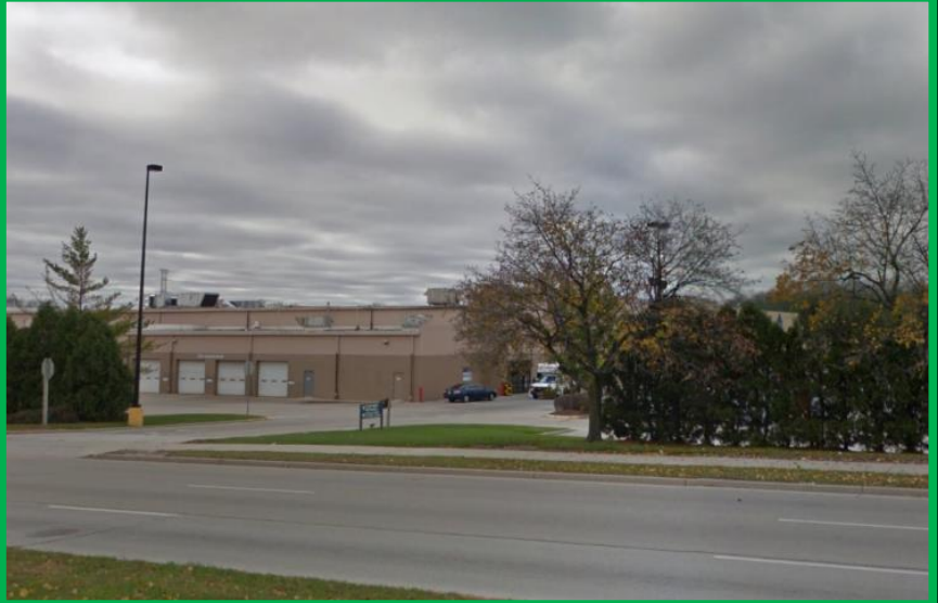
View from North 76th Street, looking west
