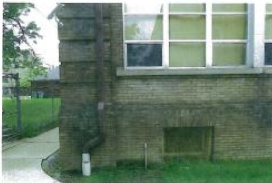
FIGURE 26: Severe deterioration of brick and mortar at northeast corner from rising damp caused by the moisture saturated and flooded basement/foundation conditions. Algae growth is also typical in this area.
