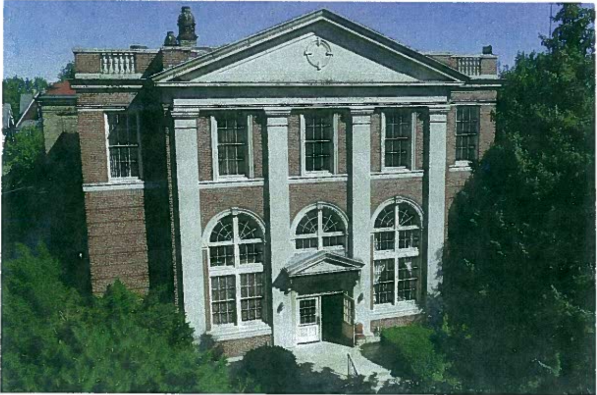
FIGURE 41: View from roof of Gymnasium/Rec Center. Wood door to be refurbished. Spalling at entry steps and crack at base of right column. Moisture infiltration through the parapet has caused spalling of the limestone details at the pediment and balustrade as well as mortar decomposition.
