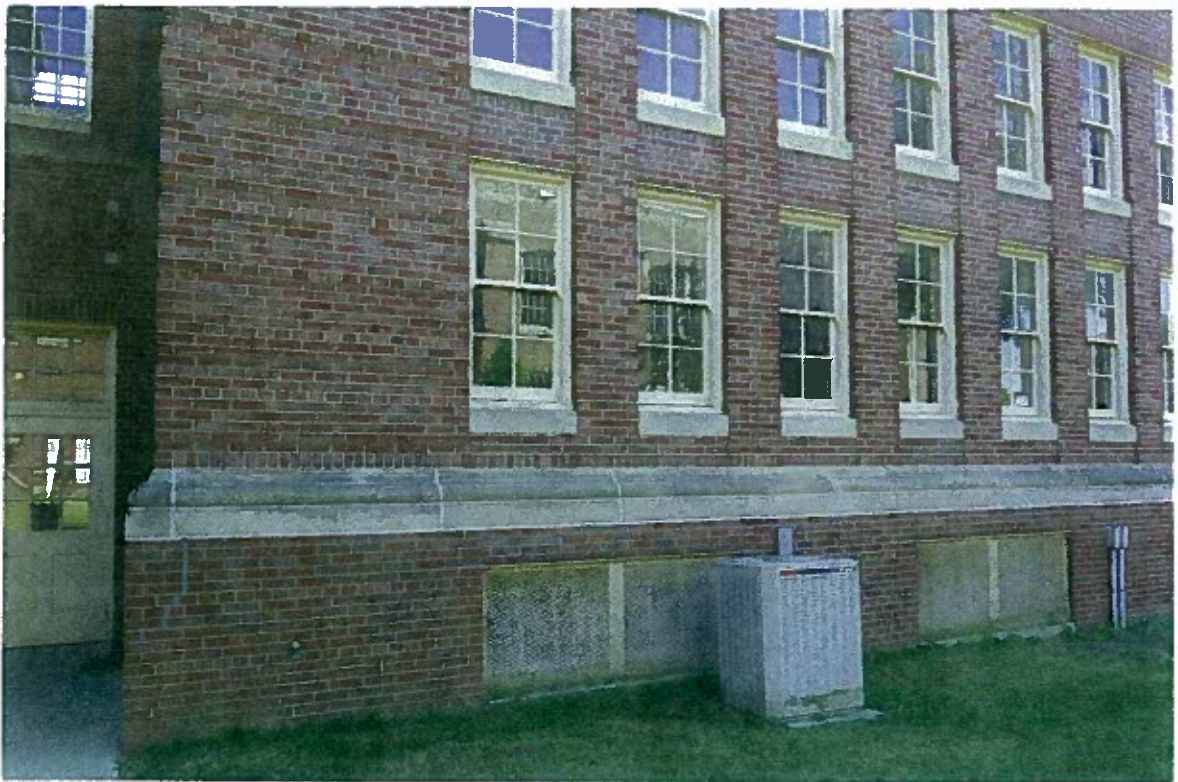
FIGURE 38: Patching at northeast corner base. Caulk at horizontal joint under water table band to be removed. Lintels at basement windows to be replaced due to corrosion and uplift causing brick damage.
