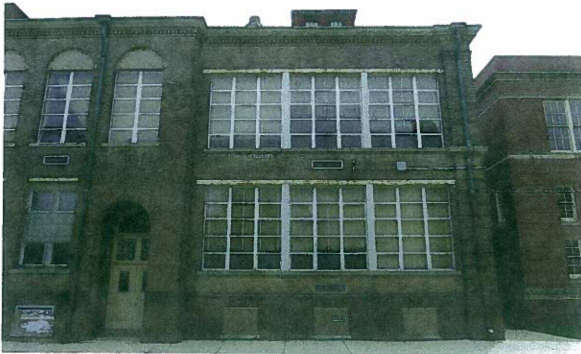
FIGURE 31: Basement windows have been bricked in. Corrosion of continuous steel lintel. Exterior door and transom to be refurbished, reglazed, paint stripped, wood primed and painted.
