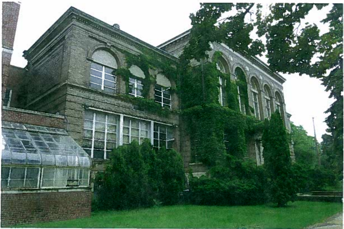
FIGURE 2: South facade. Windows other than the chapel windows above main entry are stainless steel frame and historic arch top at upper level has been filled in with a smooth brick.
