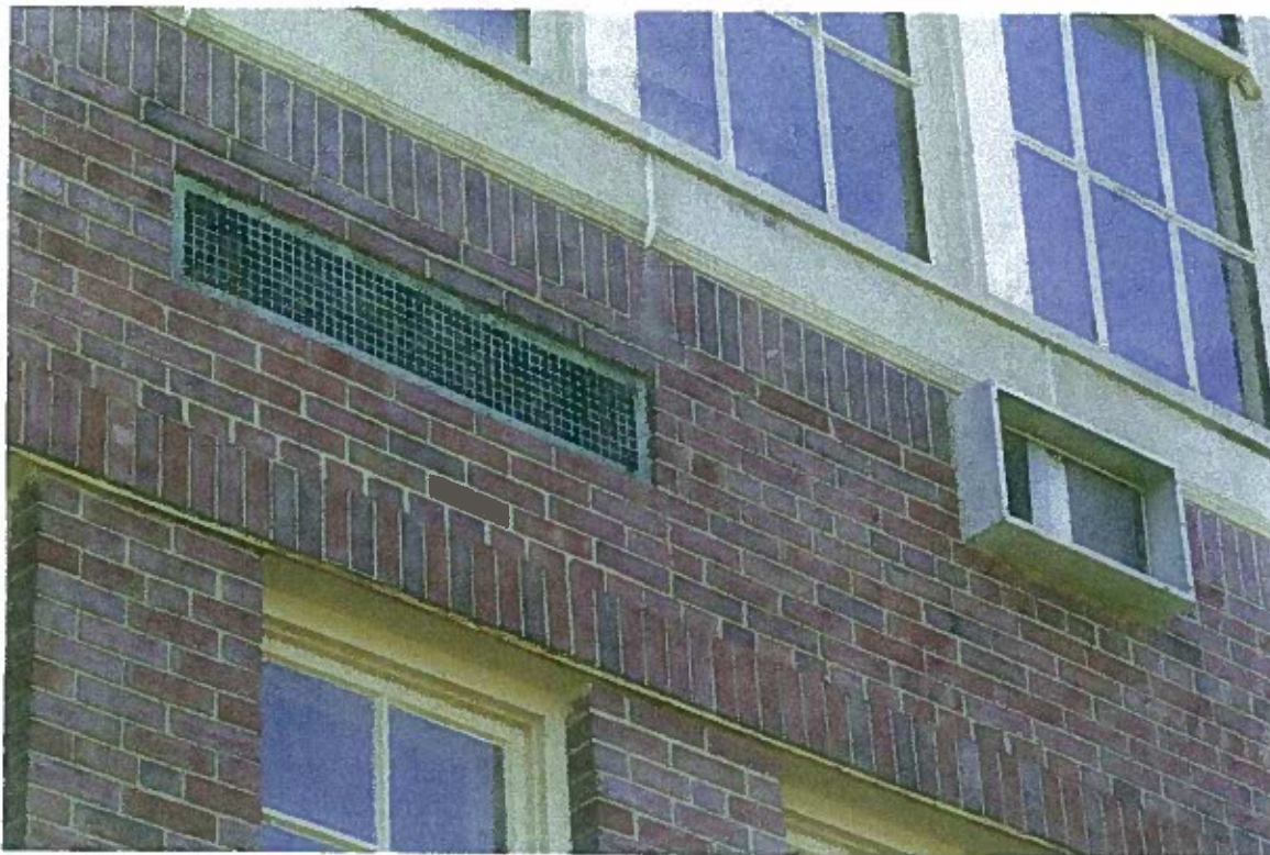
FIGURE 39: Corrosion at continuous steel lintel. Corrosion at ventilation grille and metal sleeve for missing air conditioner. Long continuous lintels can be refurbished in place.
