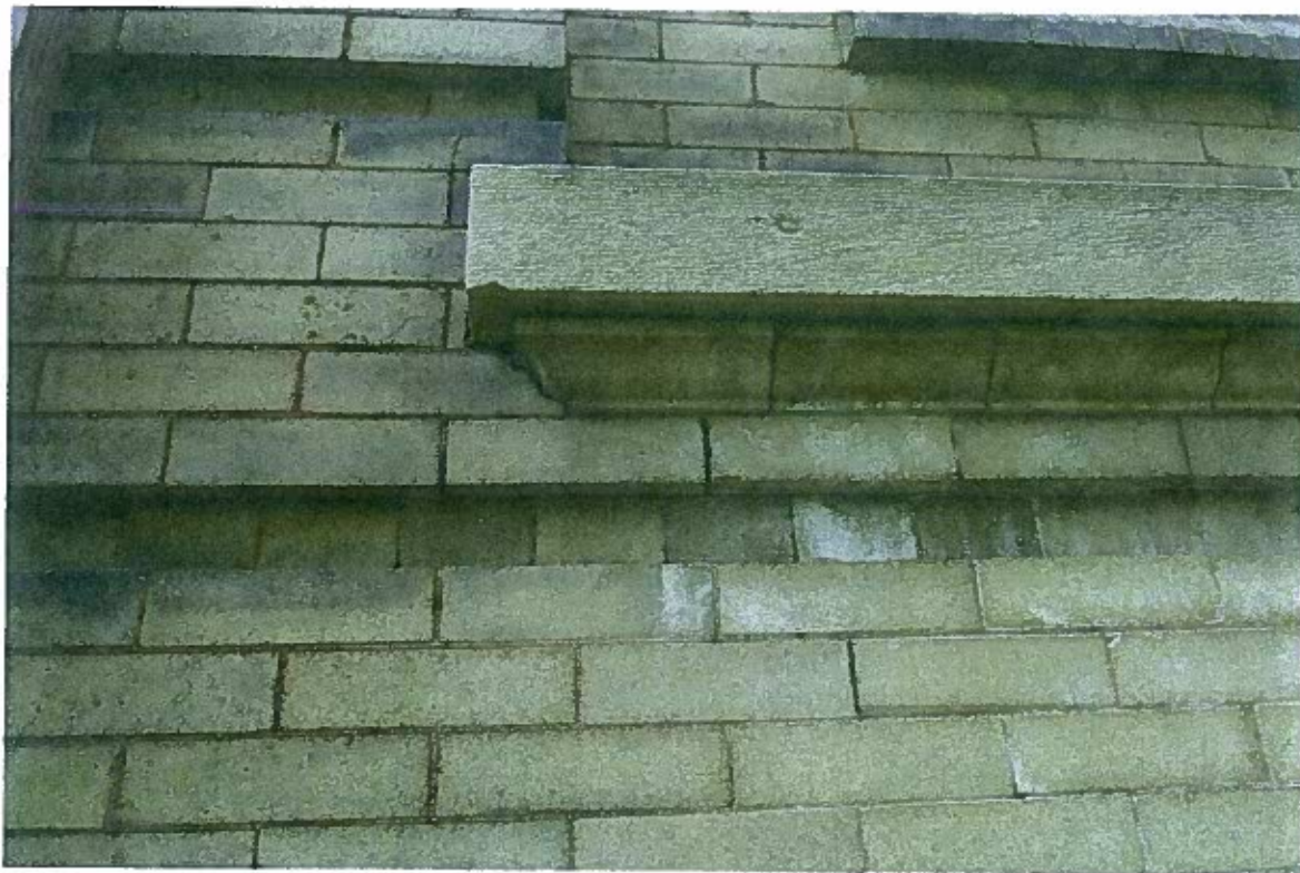
FIGURE 24: Deterioration of mortar and efflorescence below Indiana limestone sill.
