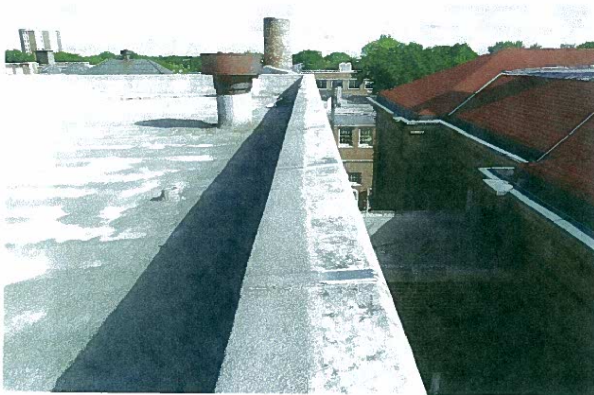
FIGURE 60: Parapet is mostly straight, but will require rebuilding due to water damage and failure of brick below. This view highlights feathering out of roofing material on top of the coping.
