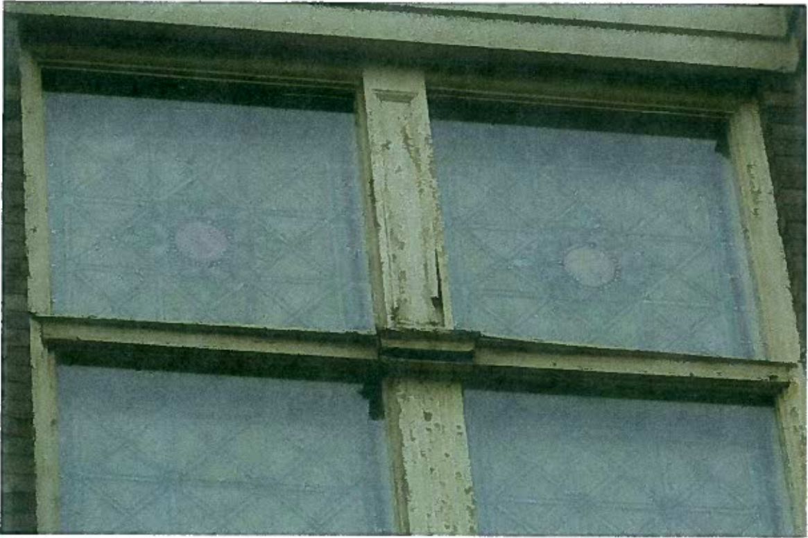
FIGURE 9: Water damage and peeling at wood window frame of chapel above main entry. Wood rot is evident.
