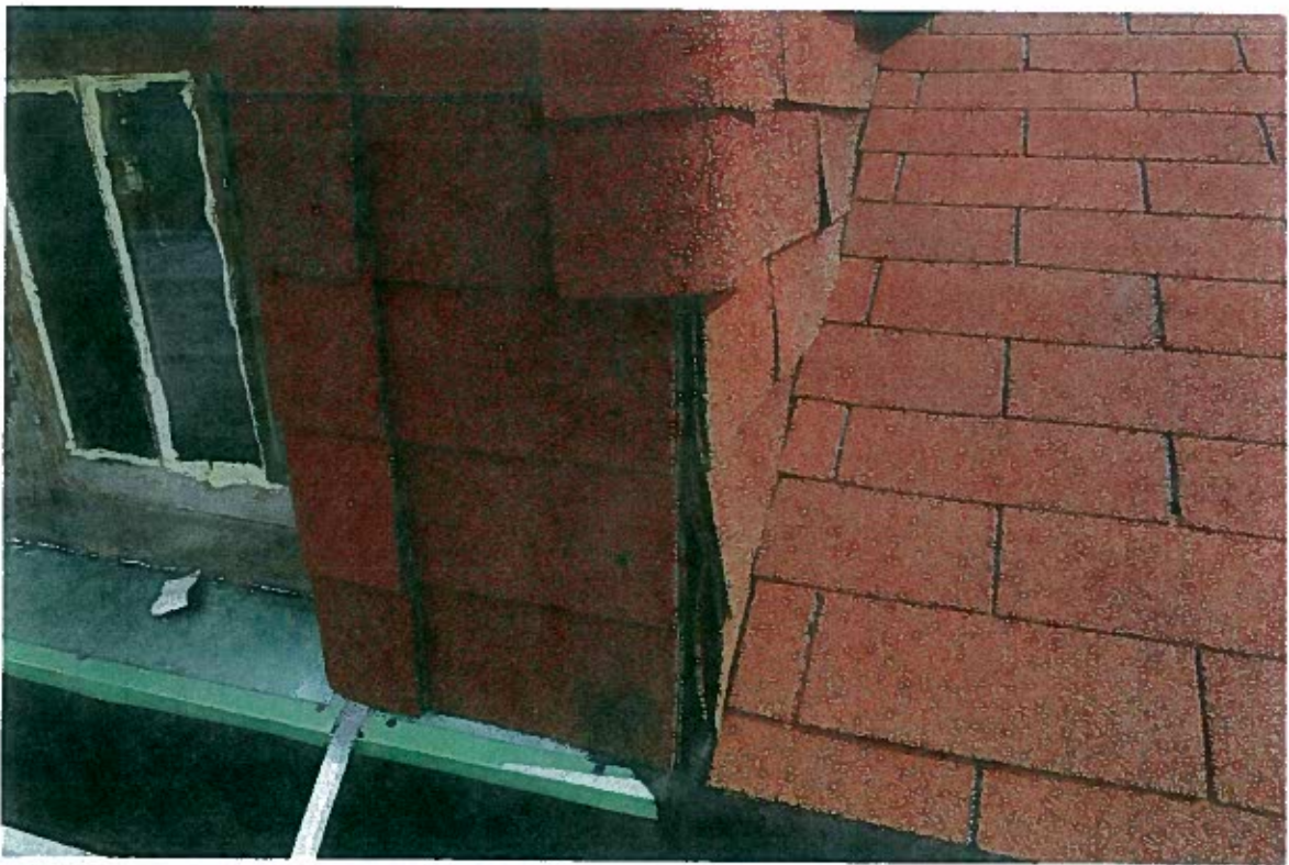
FIGURE 50: Corner shingle capping has come off, allowing water infiltration. Poor glazing and missing glass at dormer window.
