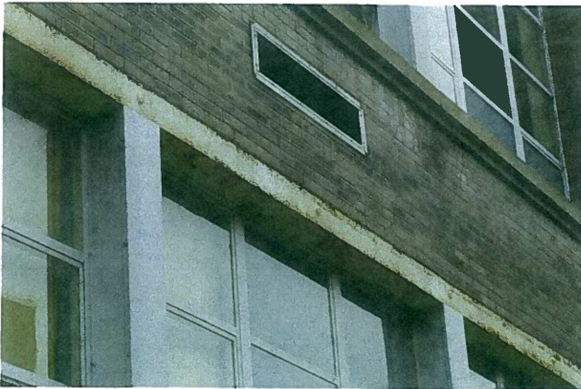
FIGURE 28: Corrosion of existing continuous steel lintel.
