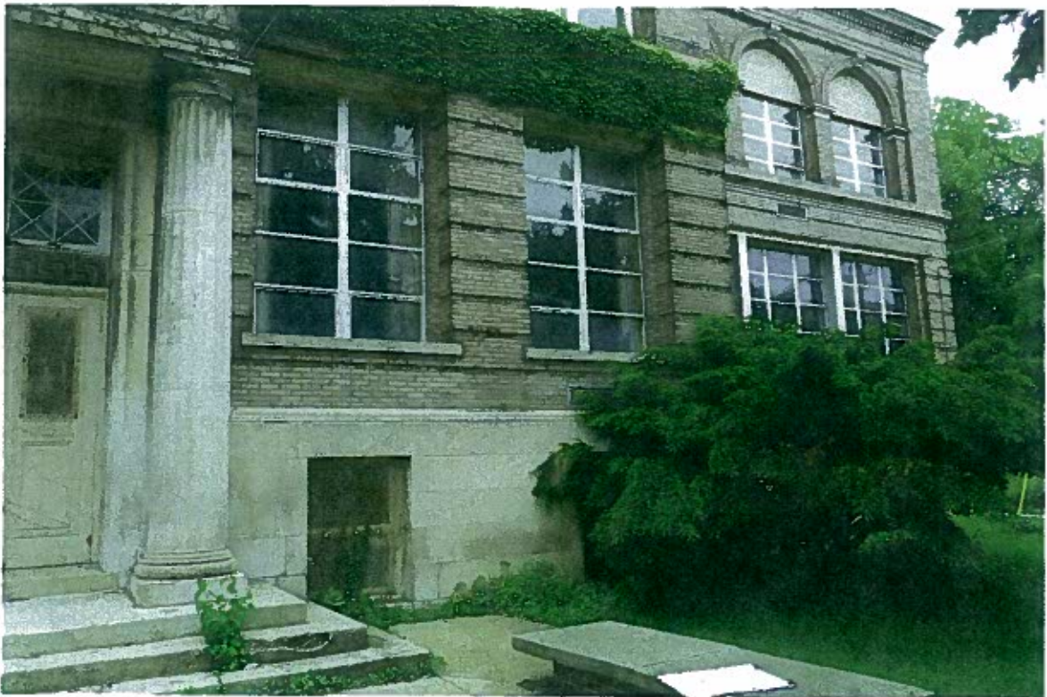
FIGURE 6: Wall area east of entry showing corrosion of lintels and spalling of concrete at steps.
