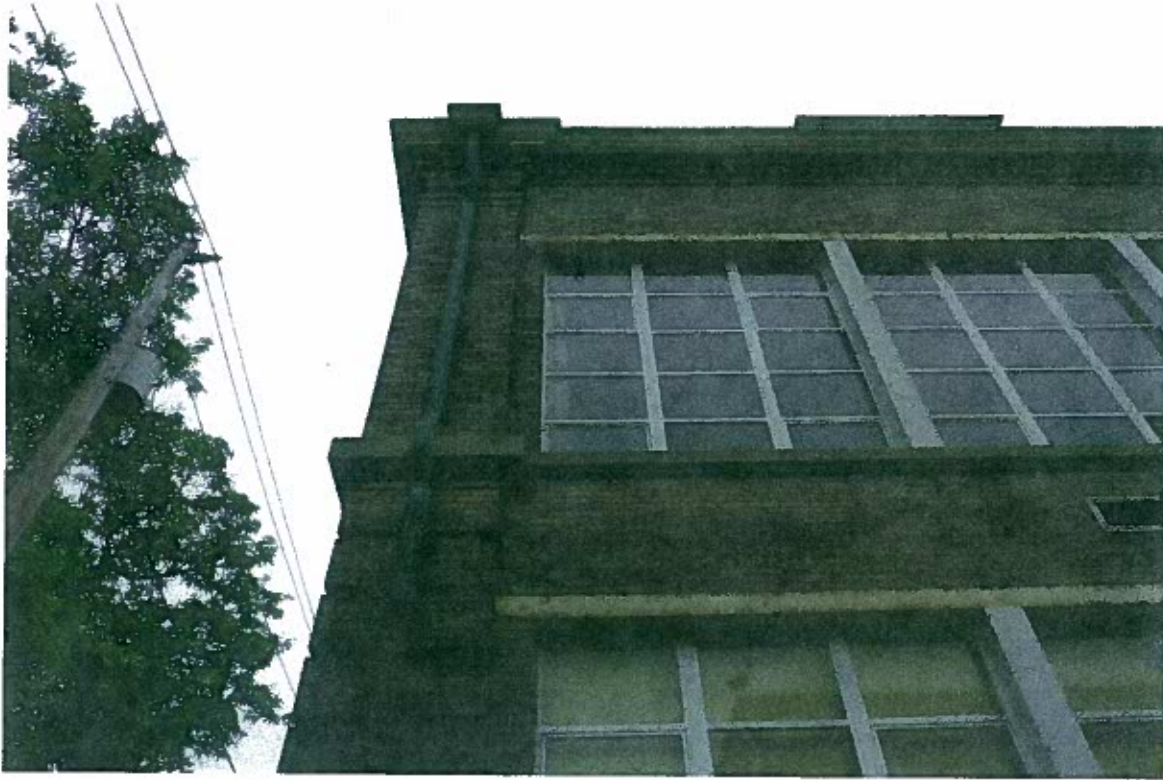
FIGURE 27: Deterioration of mortar and efflorescence below sill at northeast corner. Building was left for many years with a leaking roof that allowed moisture to saturate the walls.
