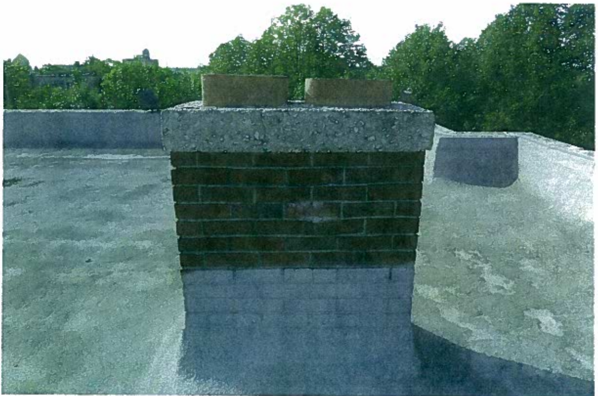
FIGURE 58: Deterioration of mortar at brick chimney and efflorescence from water infiltration. The spray-in roofing was applied up the chimney face.
