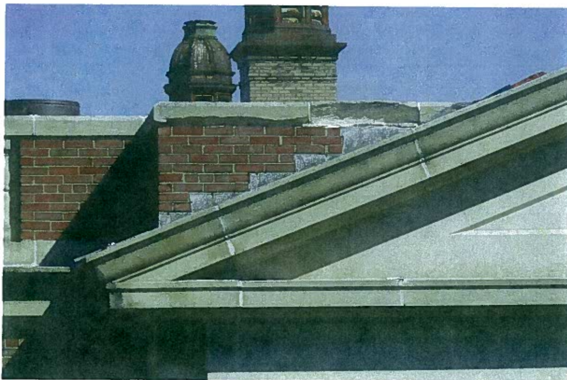
FIGURE 44: Severe spalling at Indiana limestone parapet coping and damage to brick below.
