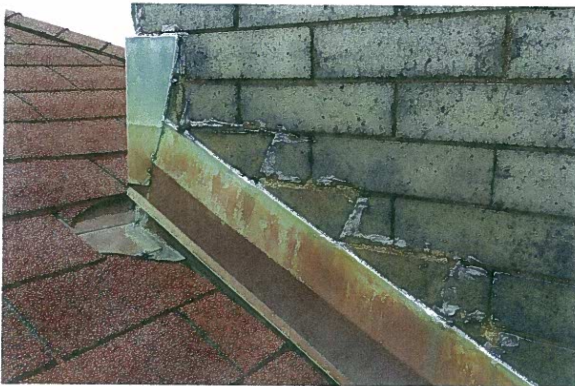
FIGURE 47: Shingle roof is in good condition. Copper flashing and counter flashing is not properly installed with a reglet and does not reach above the snowline. Tar from previous step flashing remains on the brick.
