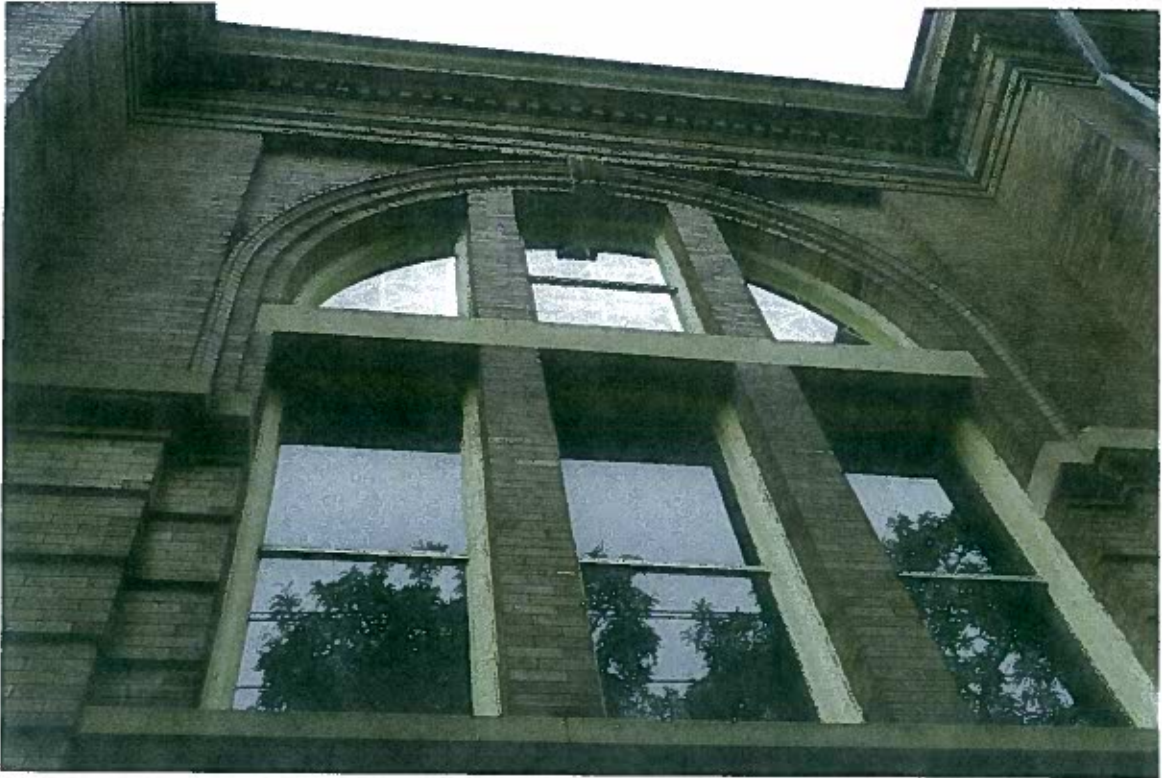
FIGURE 21: Original wood window shows water damage and peeling paint. Proposed to be stripped, primed, and painted. New glazing sealants will be installed, reputtied. Hardware is missing and will be recreated.
