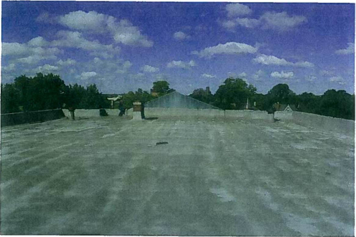
FIGURE 53: Roof looking West. Spray-on roof coating has an undulating surface and areas of ponding are visible. Beneath the spray-on roofing is spray-on foam insulation that is actively damp in all areas tested.
