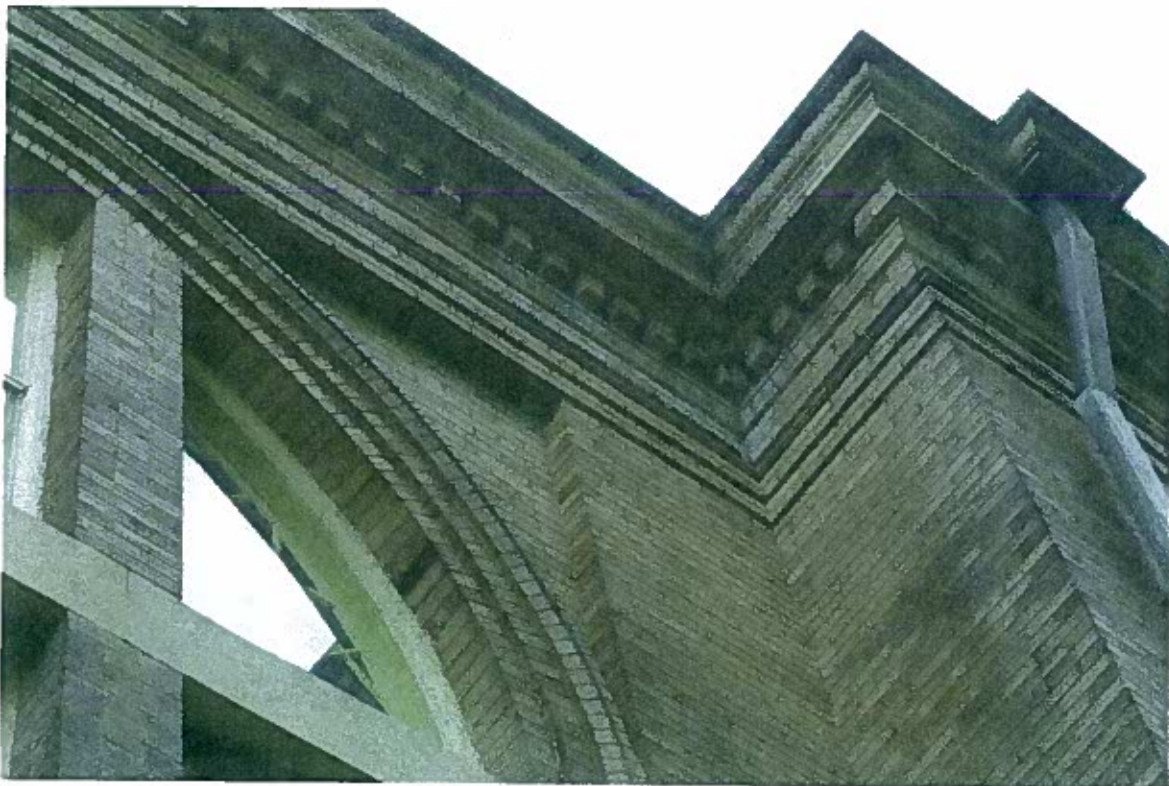
FIGURE 20: View looking up at east elevation interior corner efflorescence from prolonged exposure to moisture.
