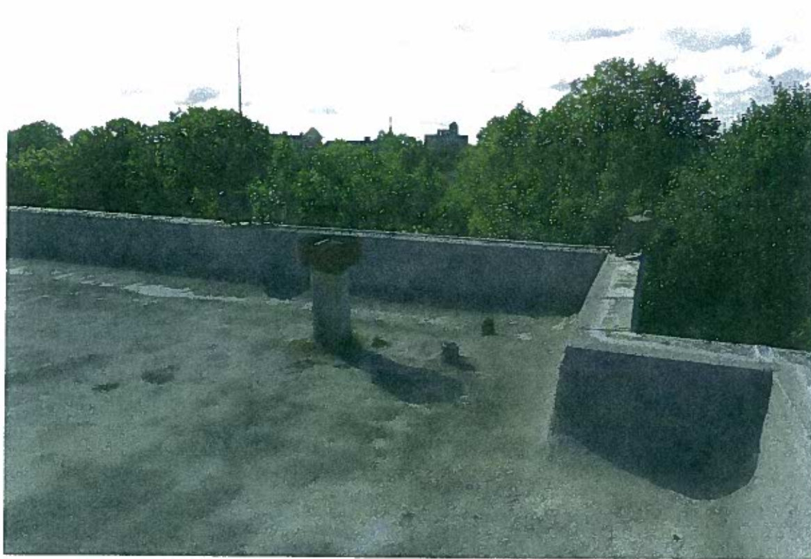
FIGURE 59: Roof ventilator and corner drain. All drains show signs of clogging. The roofing extends up to top of parapet and feathers out on top of coping. Historic roof was flashed just below coping stone and roofing applied over the flashing.
