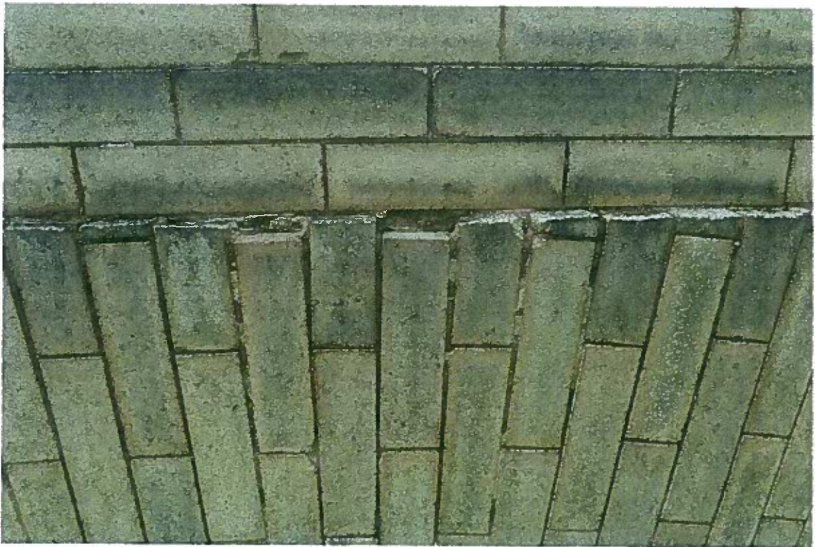
FIGURE 22: Top of jack arch at basement windows. The deterioration of mortar and spalling of brick is typical above all the basement windows on the east and north sides. Small pitting to the corners and top edges of the brick is from prolonged exposure to moisture, inappropriate pointing mortars.
