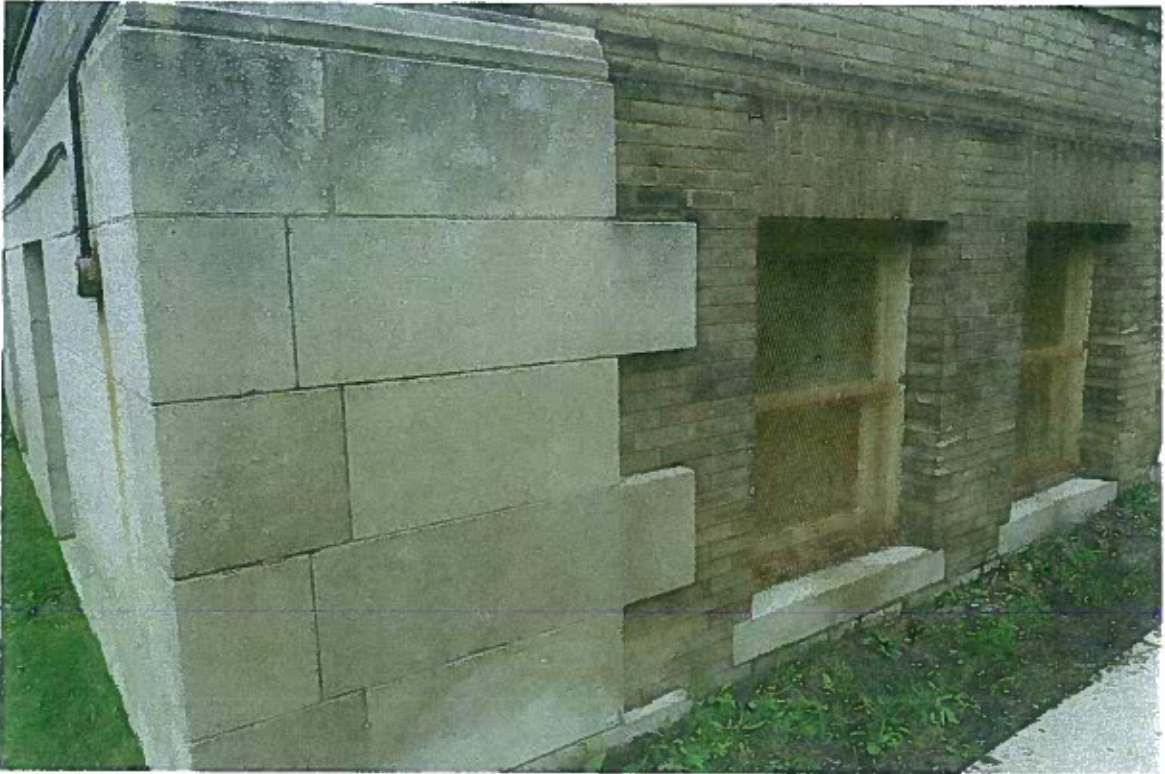
FIGURE 17: Mortar is completely decomposed in many areas of the Indiana limestone base at the south-east corner. Rising damp from the water saturated foundation has caused mortar deterioration.
