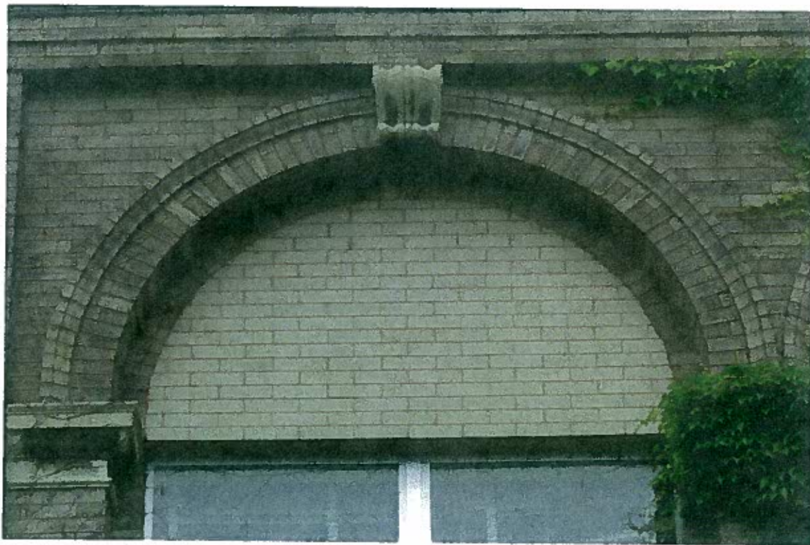
FIGURE 4: Brick infill at upper arch top windows, undated.
