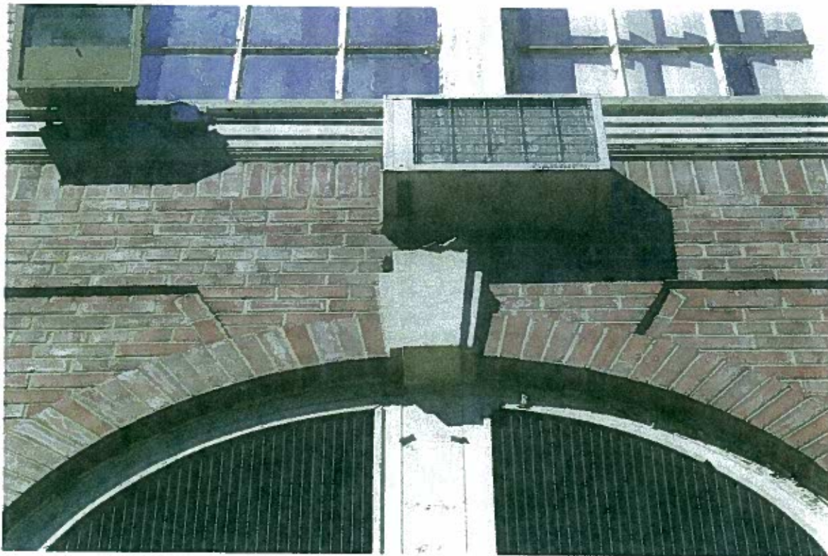
FIGURE 16: Wood windows are severely peeling. Air conditioner unit patched through wall will remain until study for future HVAC system is complete.
