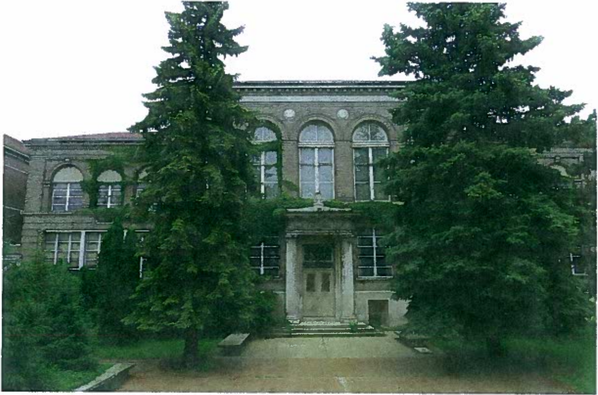
FIGURE 1: South facade and main entry. Chapel windows above main entry are wood, all others on this elevation are stainless steel frame.
