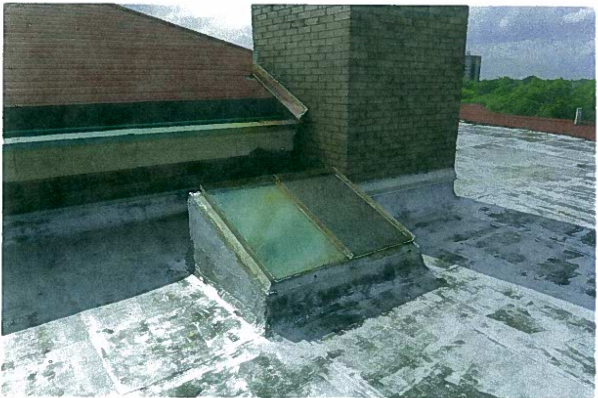
FIGURE 46: Corroded frame of skylight to attic area.
