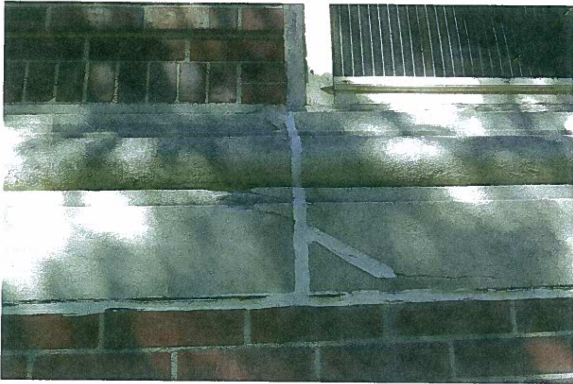
FIGURE 15: Cracking, spalling, and patches at existing Indiana limestone water table.
