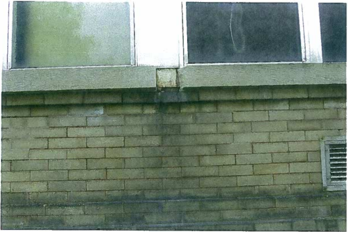
FIGURE 29: Missing section of Indiana limestone sill at a stress crack.
