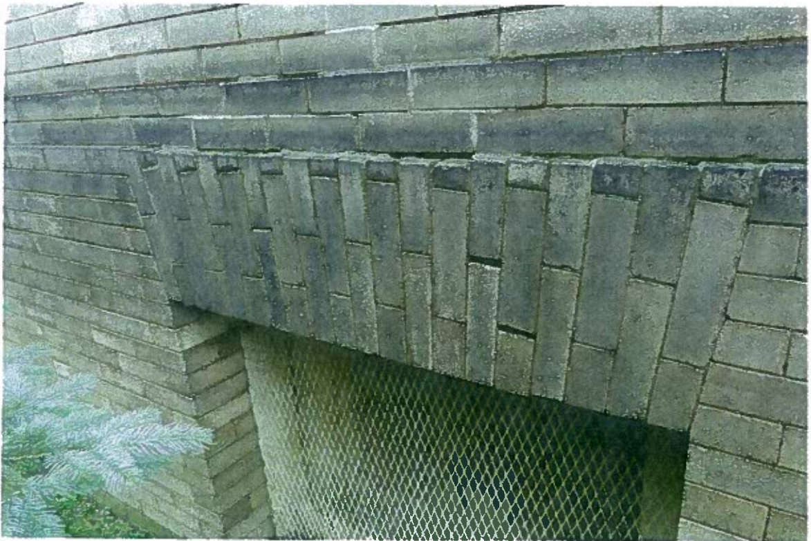
FIGURE 30: Deterioration of mortar at jack arch over basement window. Brick is slipping out of place.
