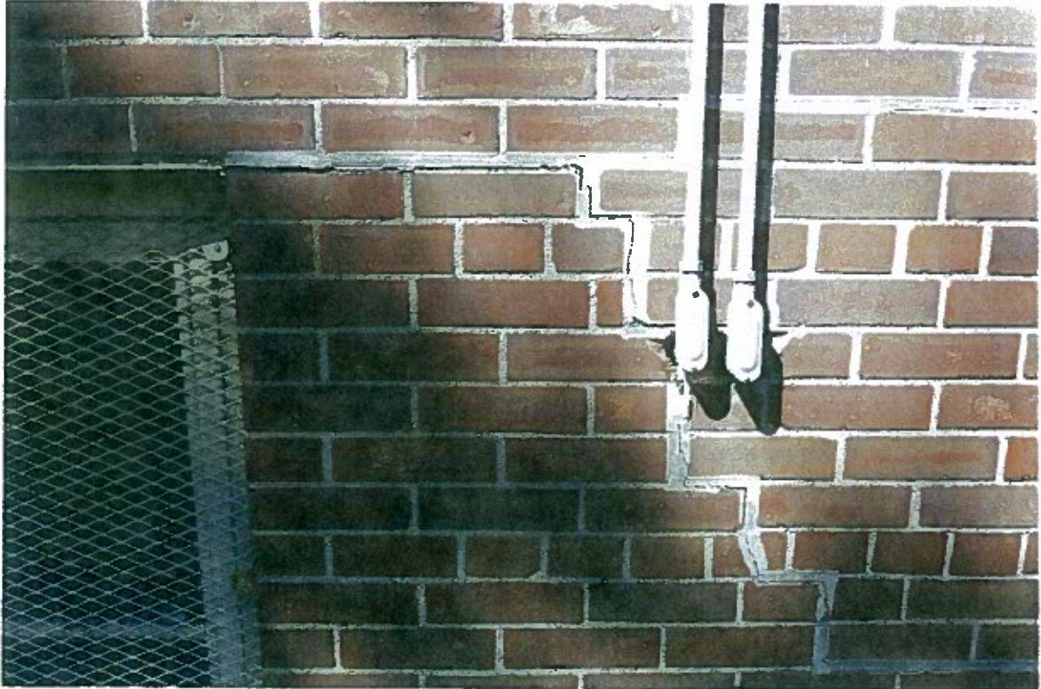
FIGURE 14: Patching evident at meandering crack from the corroded lintel uplift near a south elevation basement window.
