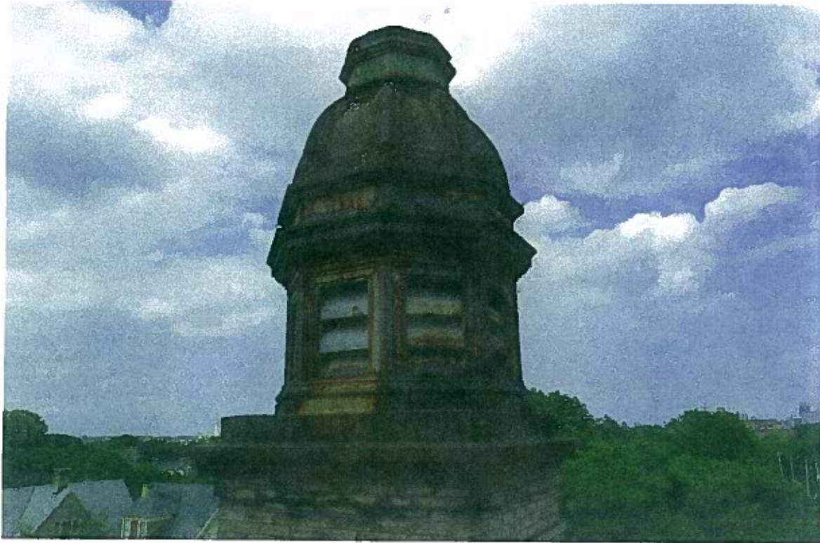
FIGURE 51: Chimney/roof top ventilators are severely corroded. Require patch replacing and removal of corrosion from entire element, then prime and paint.
