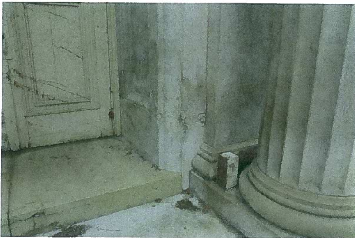
FIGURE 7: Spalling of limestone at main entry and water damage to main entry door. Efflorescence from use of deicing salts and prolonged exposure to moisture.
