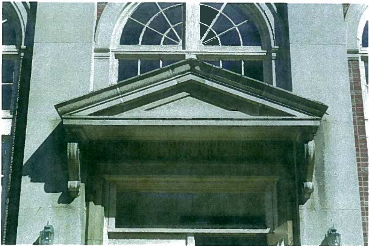
FIGURE 42: Indiana limestone canopy and inscription at main entry to Library. Indiana limestone to be cleaned.
