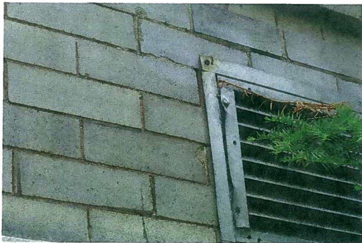
FIGURE 8: Pockets of deteriorated mortar in butter joints and drifting of brick under sill.
