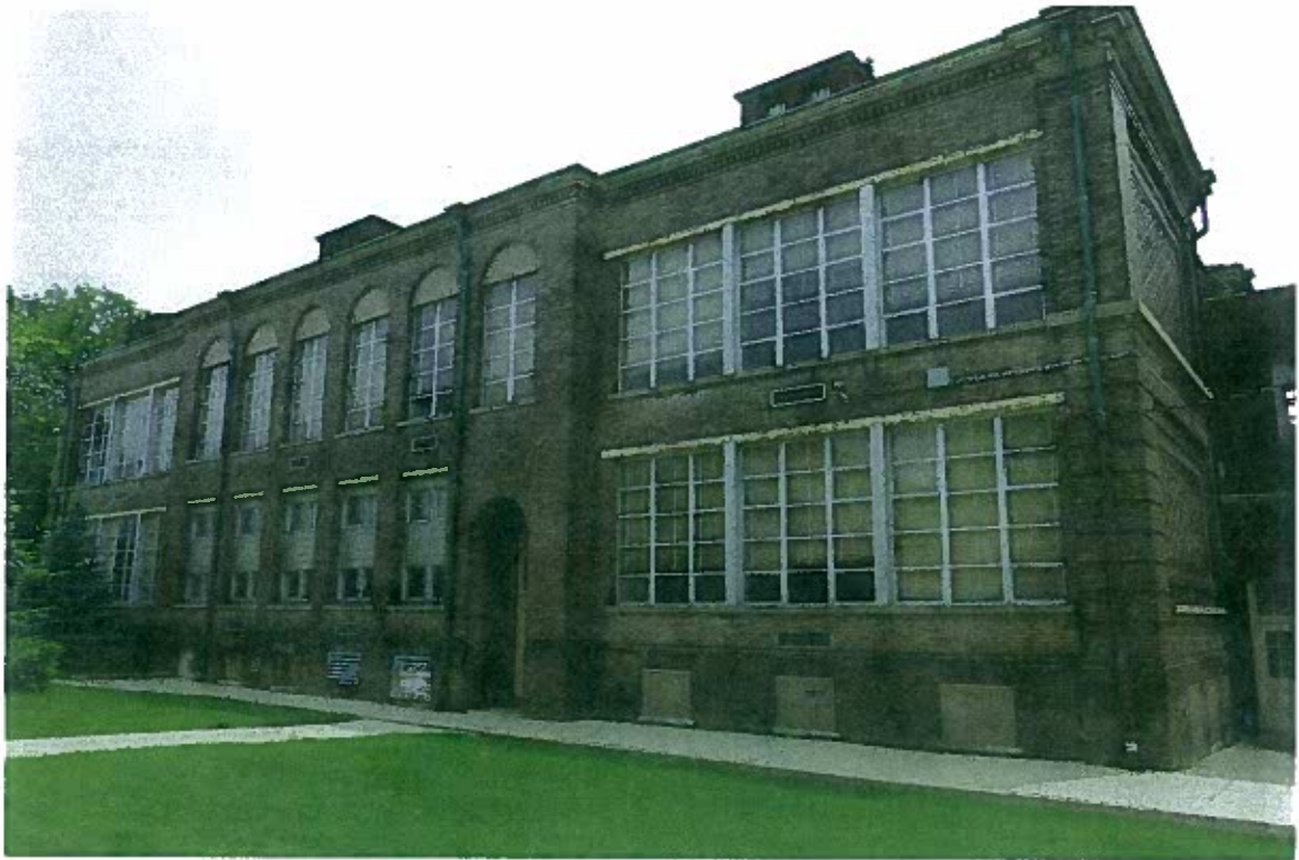
FIGURE 25: View looking southeast. Connection to Rincker Library appears at right. Discoloration at the building base due to rising damp from severe water infiltration.
