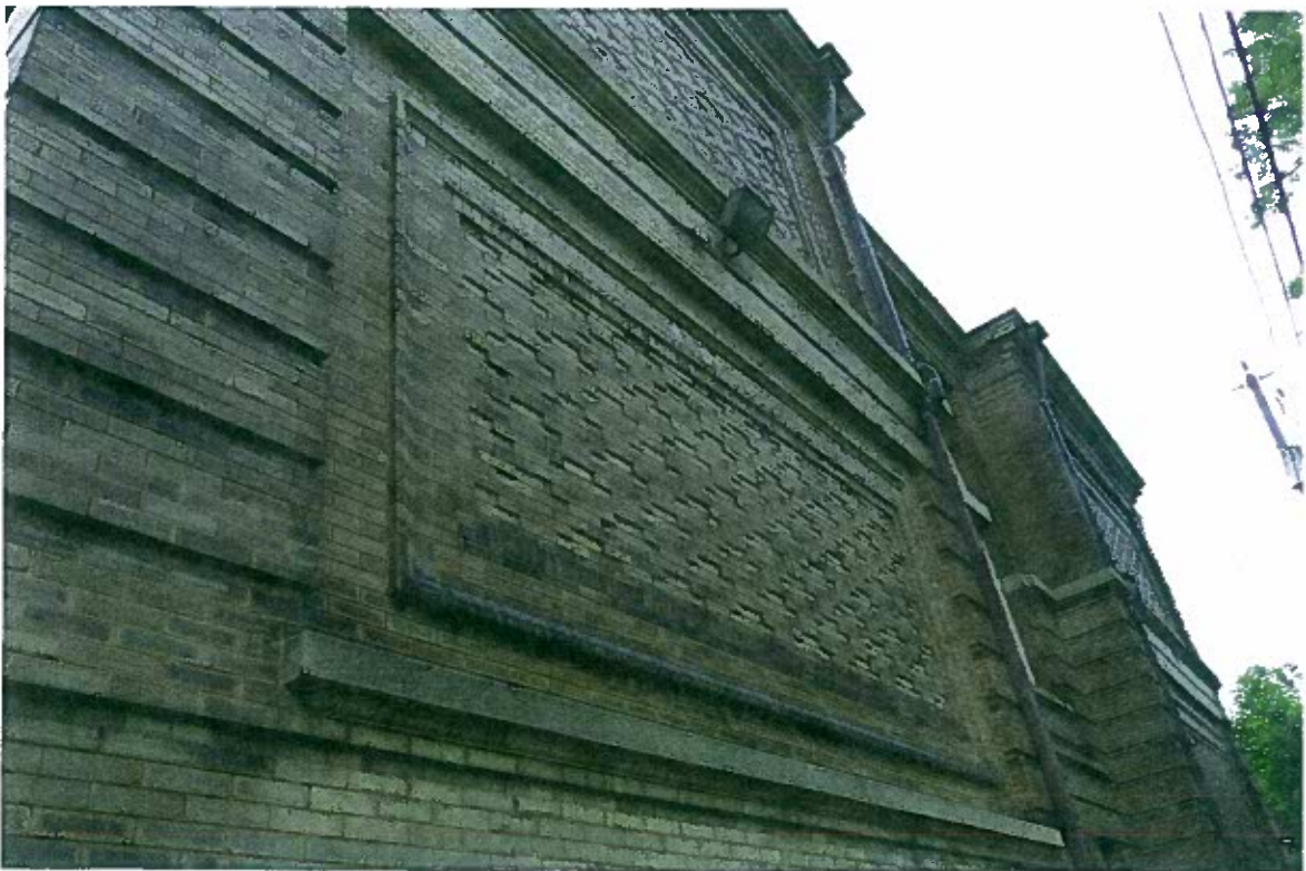
FIGURE 18: East facade showing brick details. Ironspot brick with butter joint. Projecting details courses, Flemish cross design at east and west elevations.
