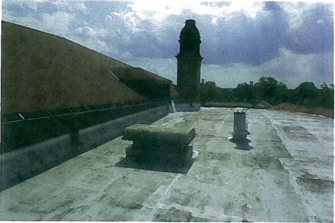
FIGURE 45: Flat roof looking due West, ventilation chimney at background. Current rubber membrane and asphalt shingle roofing is in good condition.
