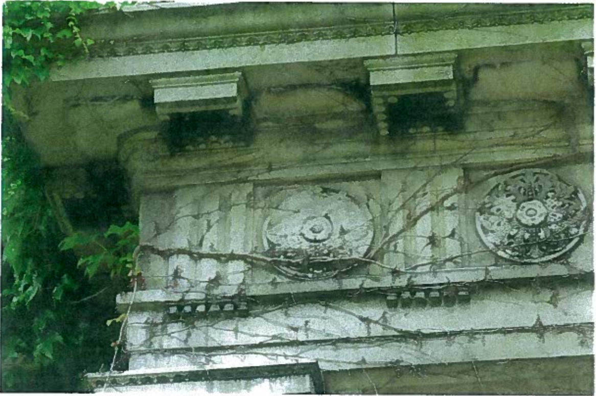
FIGURE 5: Indiana limestone at south entry exhibits moisture damage with spalling of details.
