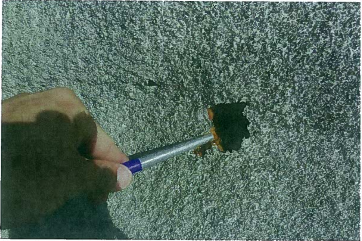
FIGURE 57: Holes in roofing expose insulation below. Insulation is actively very damp with moisture meter reading upwards of 35% WME (wood moisture equivalent).
