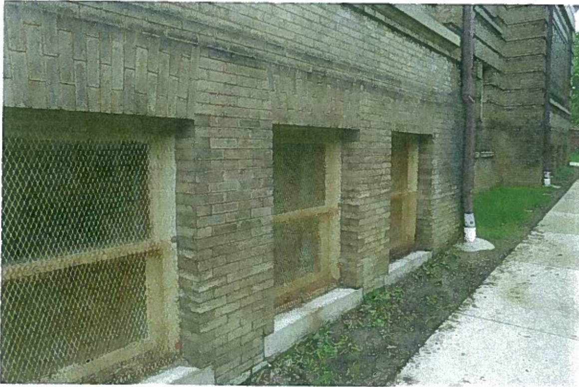
FIGURE 19: View looking north along east side showing corrosion of protective window grates.
