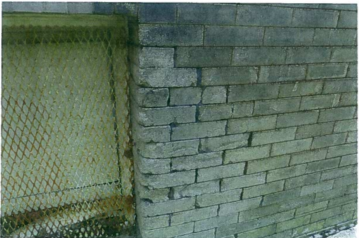
FIGURE 34: Acid etching of brick and mortar from severe moisture infiltration at window west of basement entry. Brick in this area will need to be replaced.
