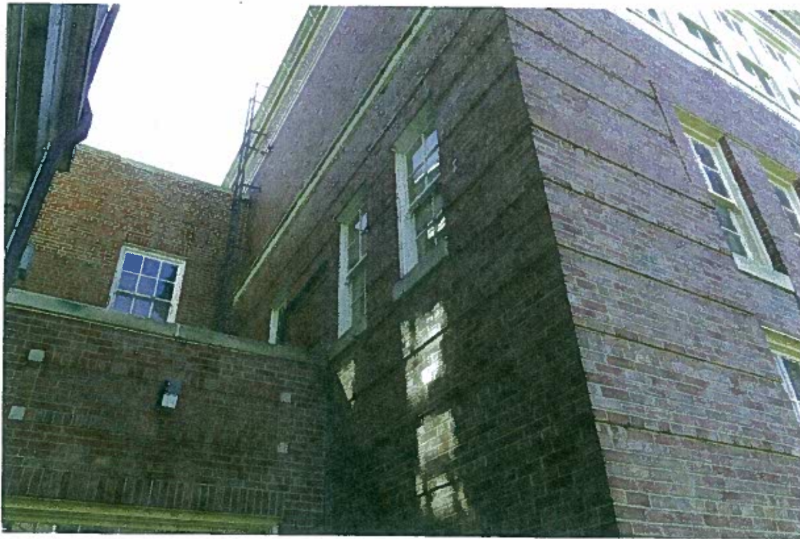
FIGURE 36: Rincker Library east elevation and connector to Albrecht Hall. Access ladder is loose at top due to masonry deterioration at parapet.
