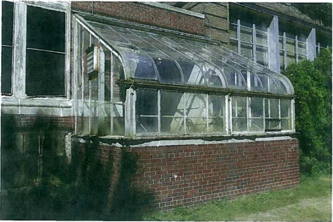
FIGURE 13: Severe deterioration to all aspects of the greenhouse addition. This greenhouse is proposed to be removed to allow for an accessible entry that would serve both buildings. The limestone sill is spalling, brick is loose (cracks are evident), and mortar is decomposed. There is no modern use for this educational greenhouse within the proposed reuse plans.
