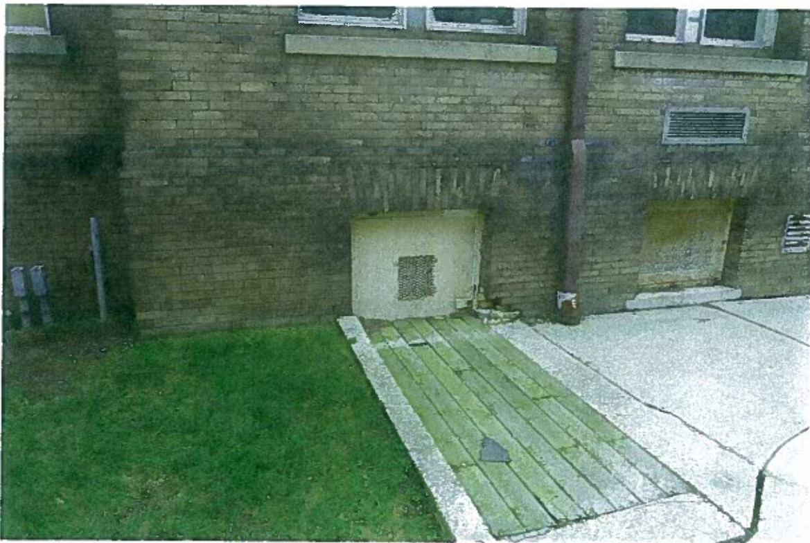
FIGURE 32: Deterioration of mortar around basement exterior entry. Water penetrates boards and collects at bottom of steps leading down to this door, then enters the building below door.
