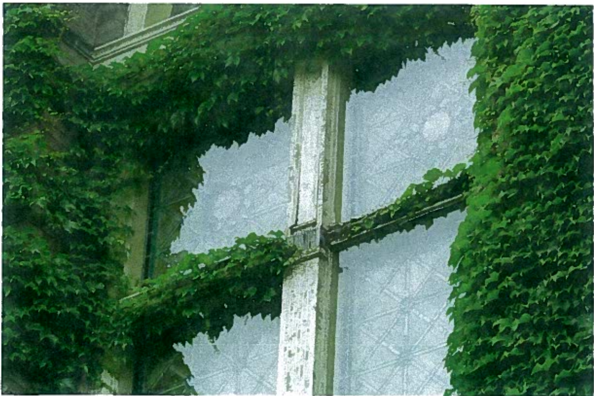
FIGURE 10: Water damage and peeling at wood window frame of chapel above main entry.
