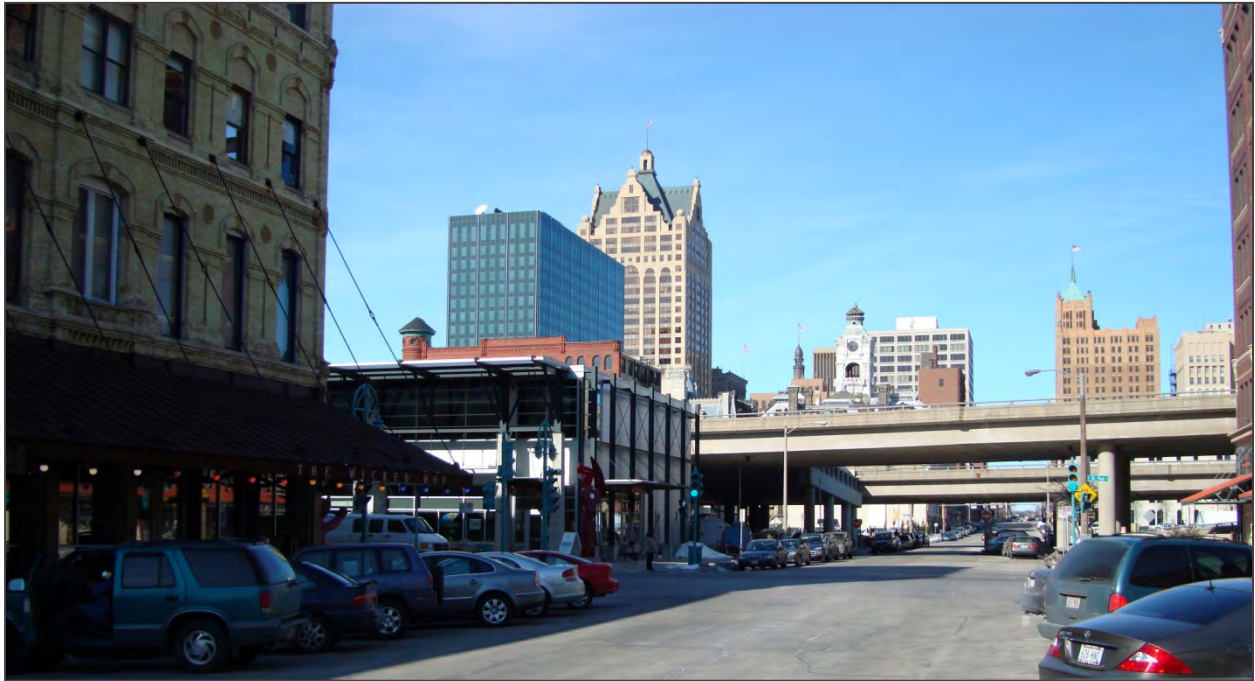
The Public Market is located in the Third Ward District. This picture shows how the Interstate 794 bridges are a prominent part of the landscape. Image: HNTB Corporation
