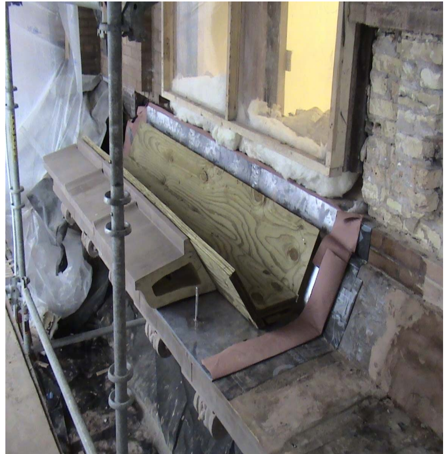
8 th floor Gutter Mock-up
