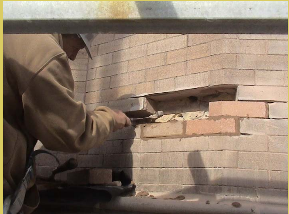
Conditional brick replacement.
