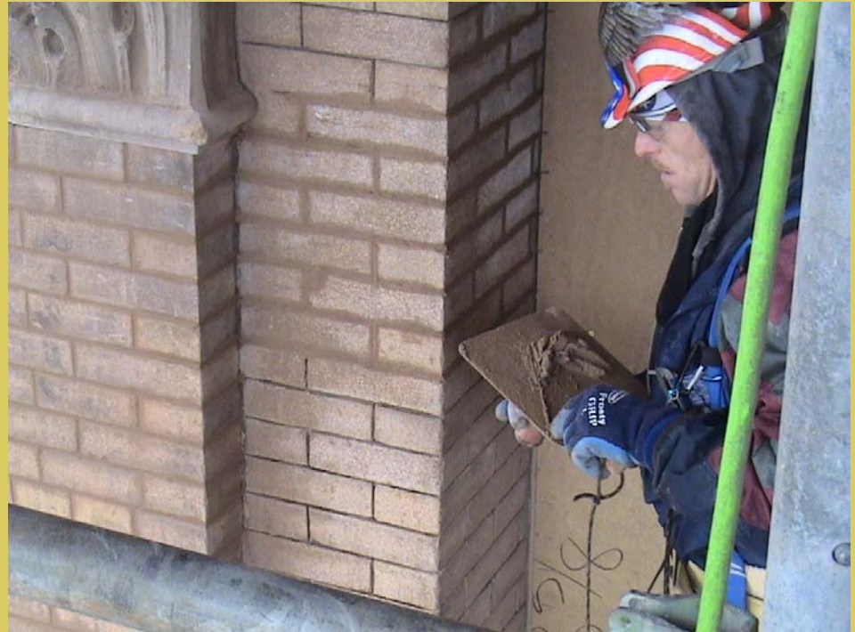
Pointing of existing brick.
