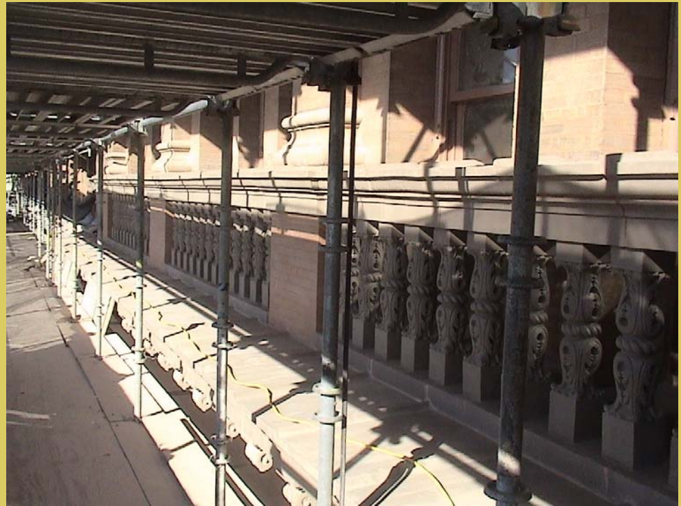
New terra cotta balustrades on east side of 8 th floor
