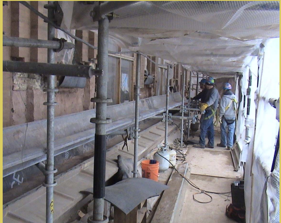
Continued soldering of lead-coated copper rain gutter.
